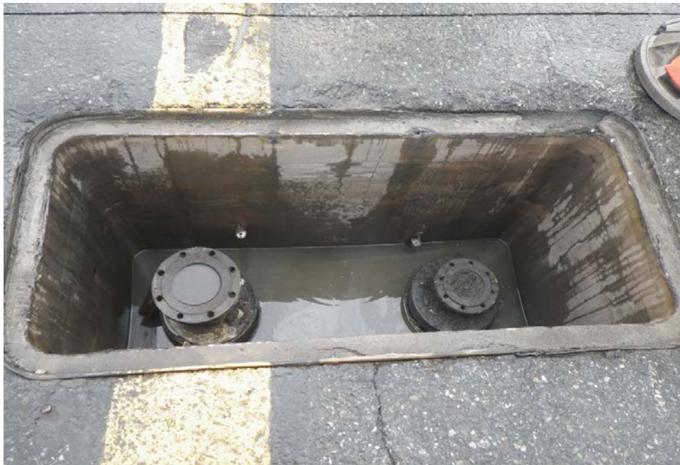
Photograph 2: View inside vault Date: 8/16/2017
