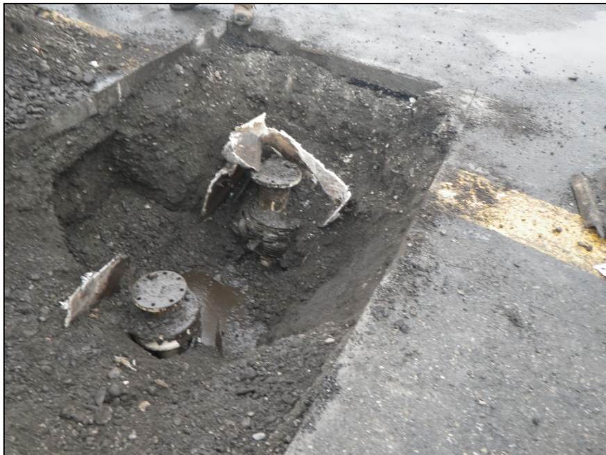
Photograph 4: Bottom of vault removal Date: 8/16/2017
