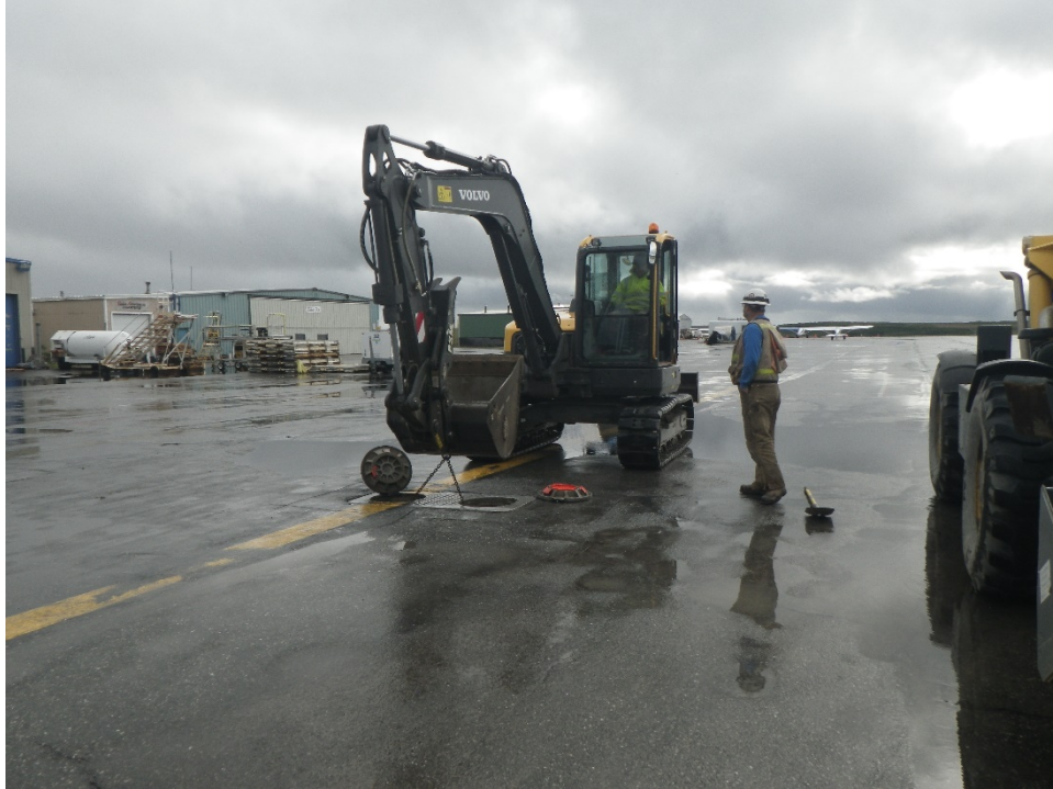
Photograph 1: Removing hydrant lid Date: 8/16/2017
