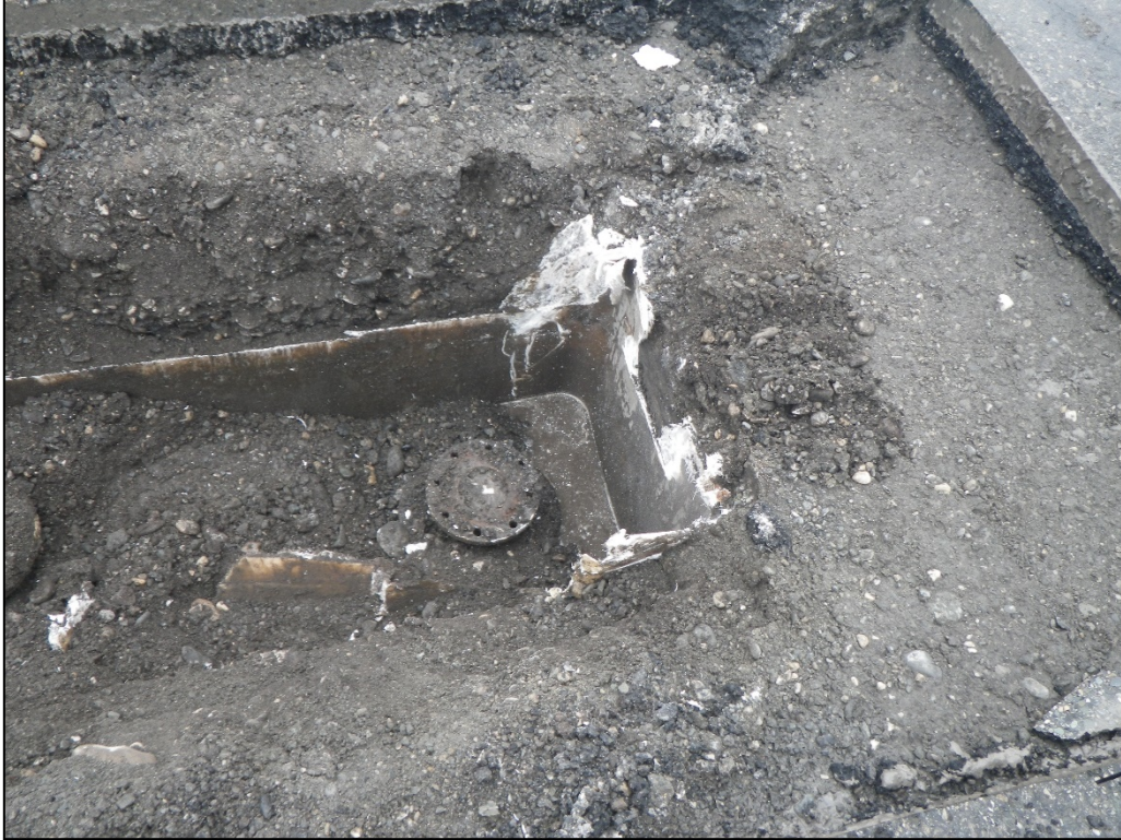
Photograph 3: Vault removal Date: 8/16/2017
