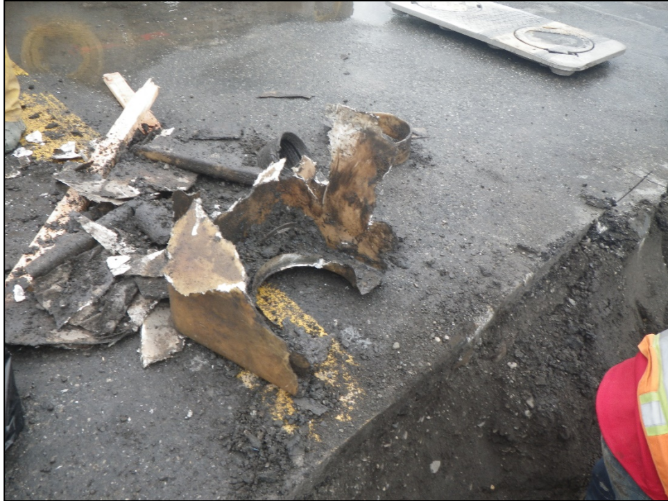
Photograph 5: Bottom of vault removed Date: 8/16/2017
