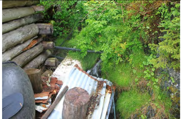
Photo showing CD4 located behind the equipment shed.
