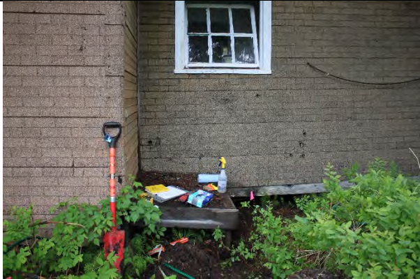
Photo showing the location of the test pit advanced at the woodshed structure (WS1).
