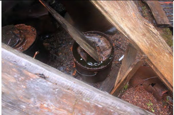
Bucket containing grease found inside the collapsed pulley house.
