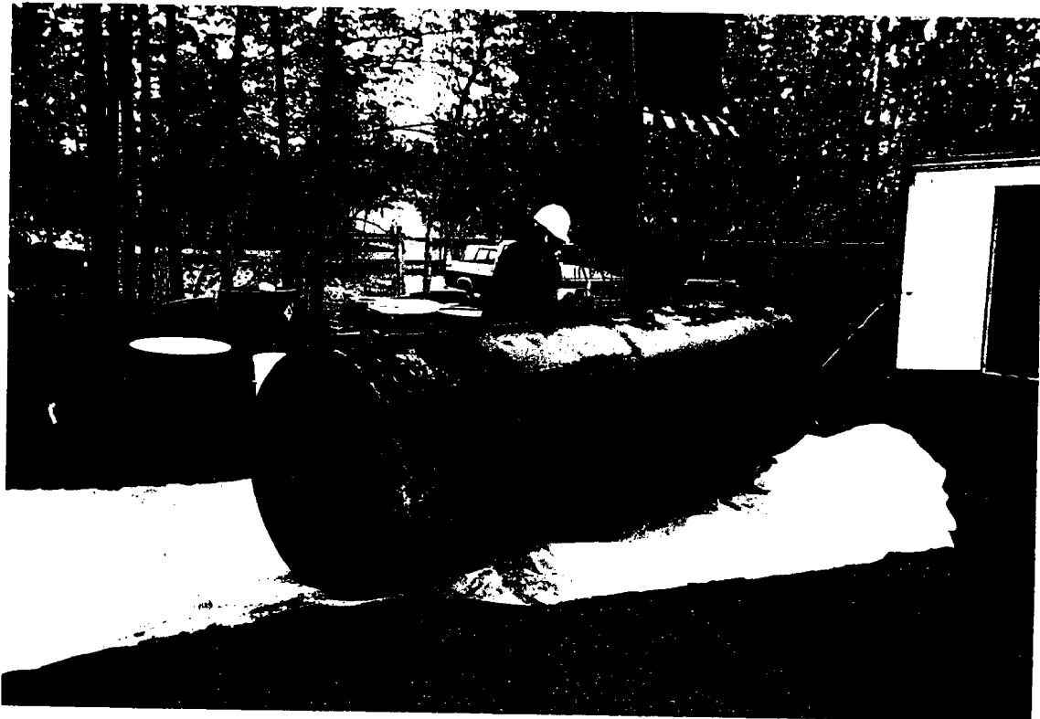
Photo 6. Used oil tank after removal.
