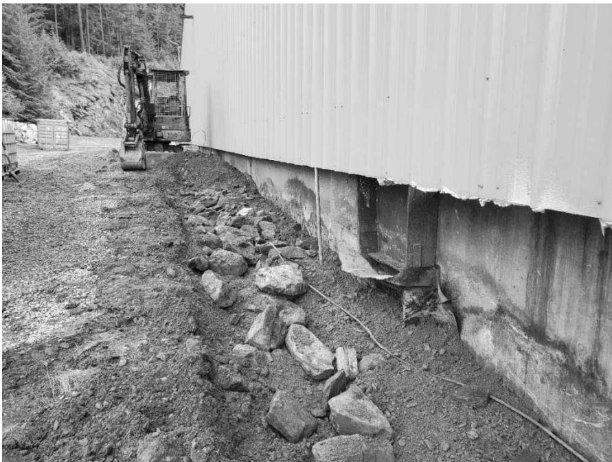
Photo 10: First round of excavation in DU3 (CSB North). Large rocks were sorted and placed back in the trench.
