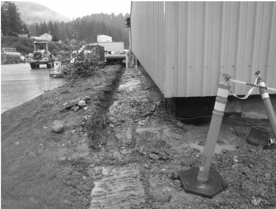
Photo 12: Completed first round of excavation in DU3 (CSB Northeast).
