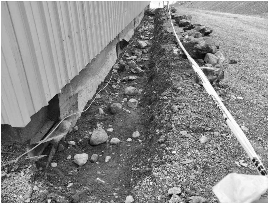
Photo 16: The completed second round of excavation in DU3 (CSB North).
