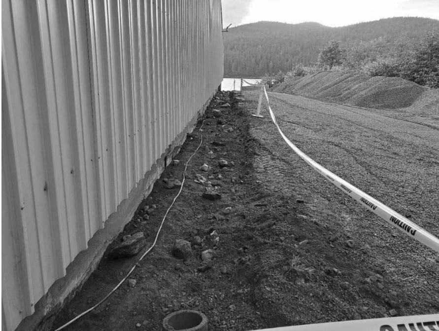
Photo 11: Completed first round of excavation in DU3 (CSB North).
