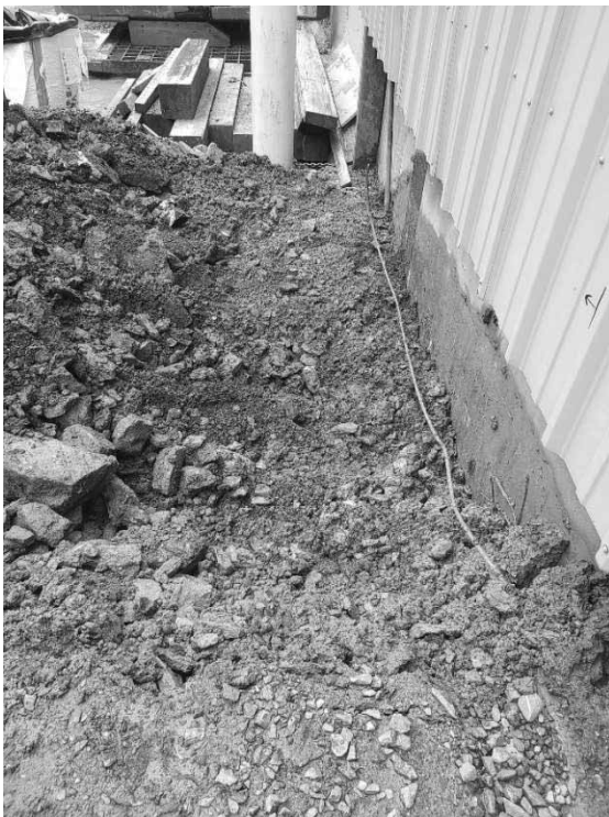
Photo 18: Additional excavation on the northeast side of CSB in May 2021.
