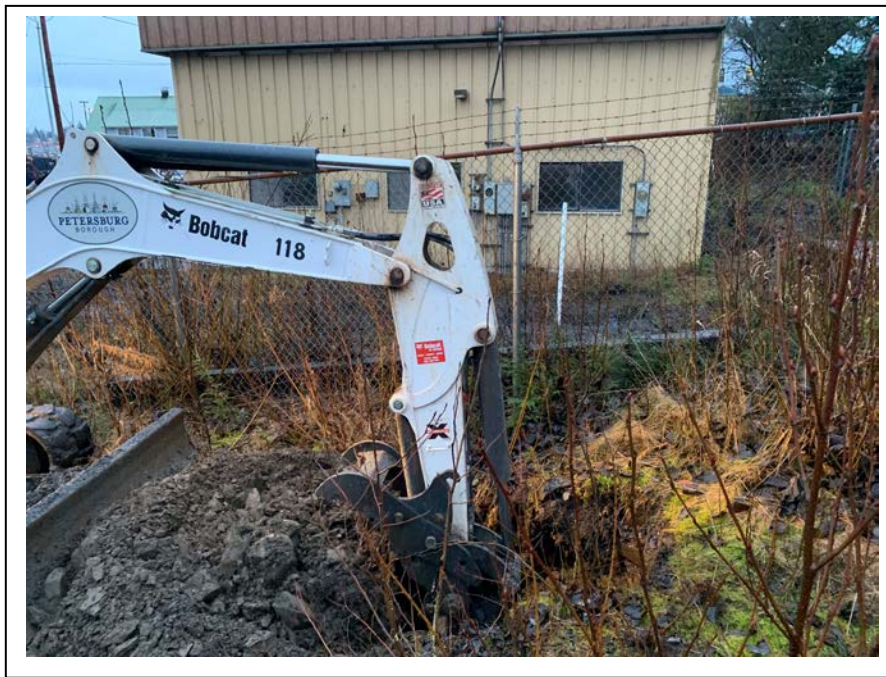
Photo 3: Looking east at the advancement of Test Pit TP8. (December 17, 2019)
