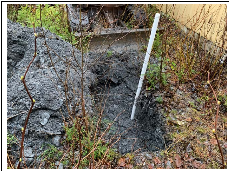
Photo 4: Looking west at Temporary Well TMW3 within Test Pit TP3. (December 17, 2019)
