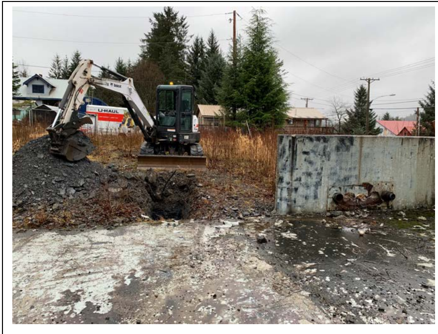
Photo 1: Looking west from the former tank farm containment area at the advancement of Test Pit TP2. (December 17, 2019)
