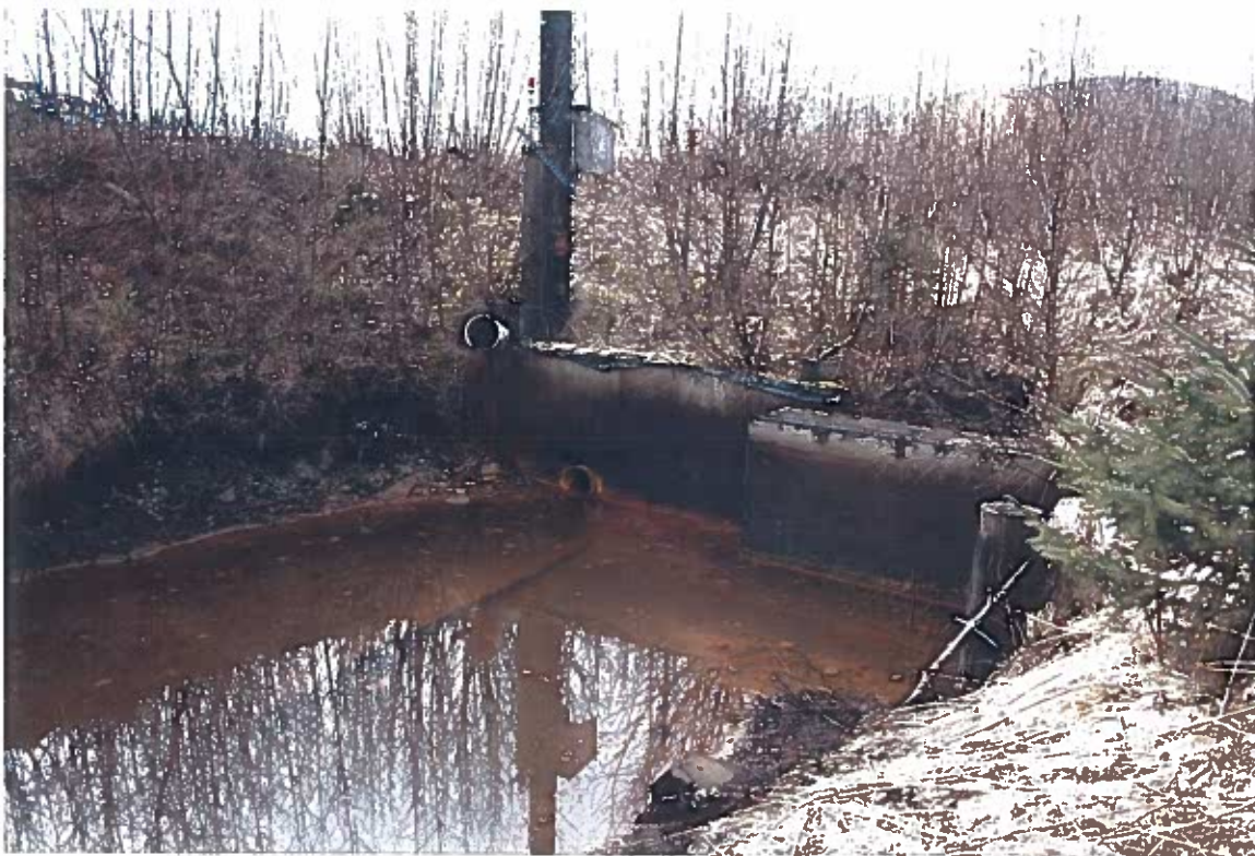
Photo #26: 3/26/12 view looking southwest at the Wrangell Lumber mill's oil/water separator inlet (arrow) and its dam structure. An approximately 1'-thick black soil ring was observed along the sides of the pond, where NORTECH's sample #SP1 had high DRO and RRO levels of 3,350 mg/kg and 15,600 mg/kg.
