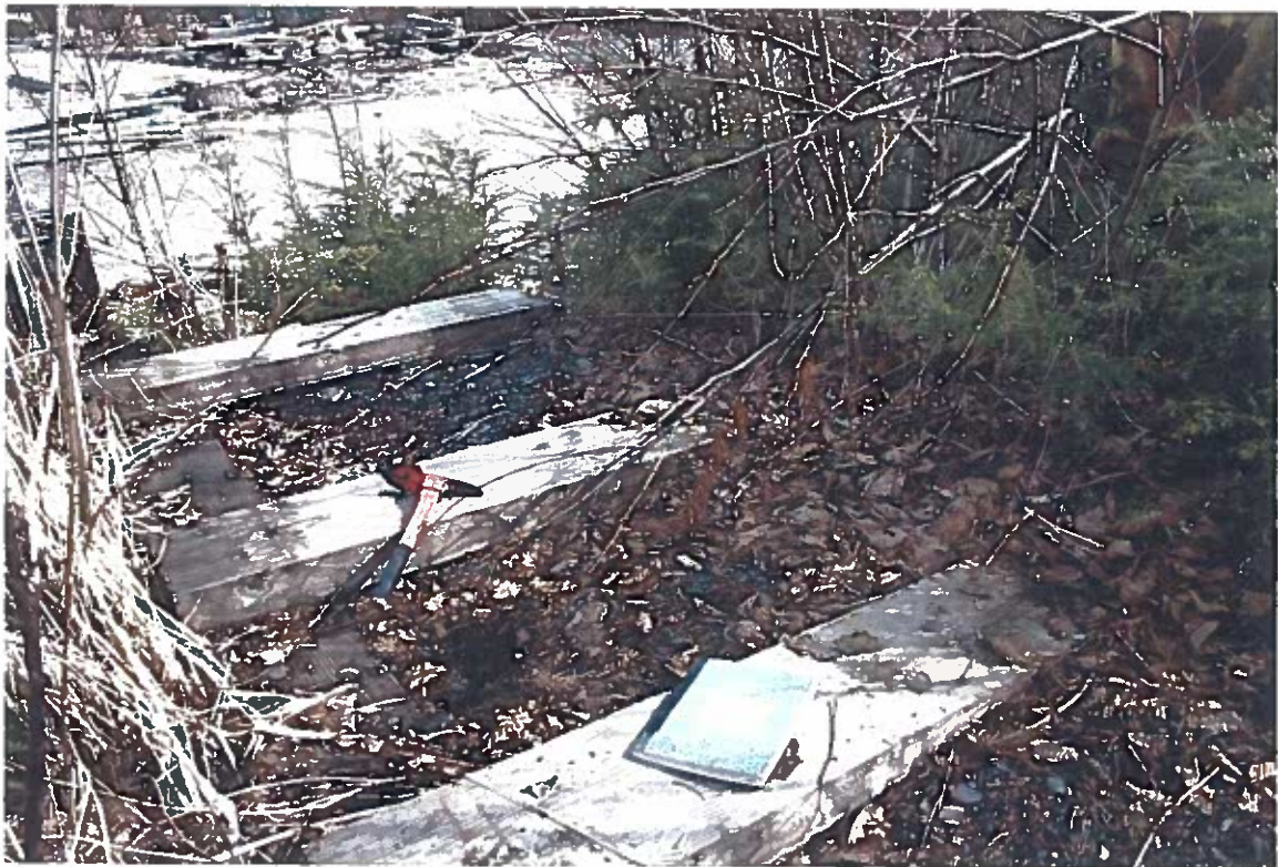
Photo #10: 3/26/12 view looking northeast across the Wrangell Lumber fuel depot's former 1,000-gallon highway diesel tank, where no signs of oil-stained soil were found.
