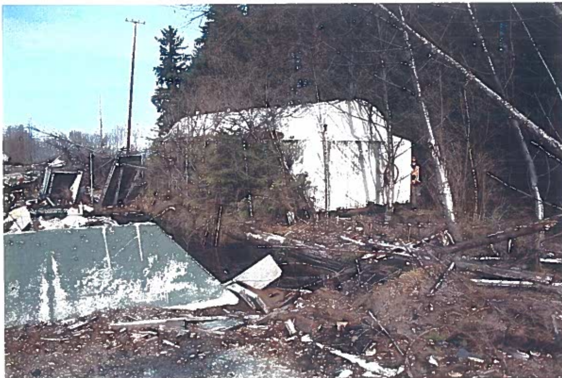
Photo #3: 3/26/12 view looking northwest at Wrangell Lumber's 20,000-gallon former generator diesel oil tank, along the north side of the mill site. See photo below.
