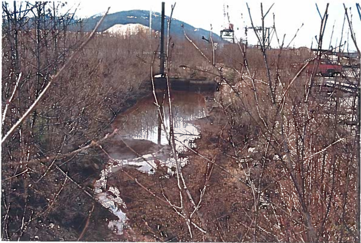
Photo #25: 3/26/12 view looking west at the Wrangell Lumber oil/water separator pond, see next 2 photos.
