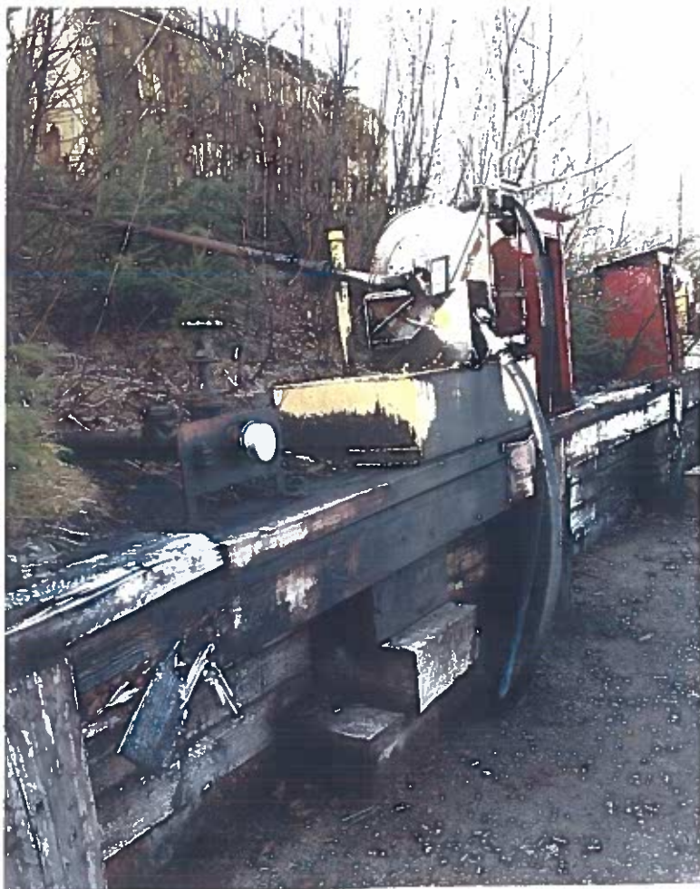
Photo #7: 3/26/12 closer view of the Wrangell Lumber fuel depot's diesel oil dispenser, showing black oil stains extending into the soil behind the bulkhead.
