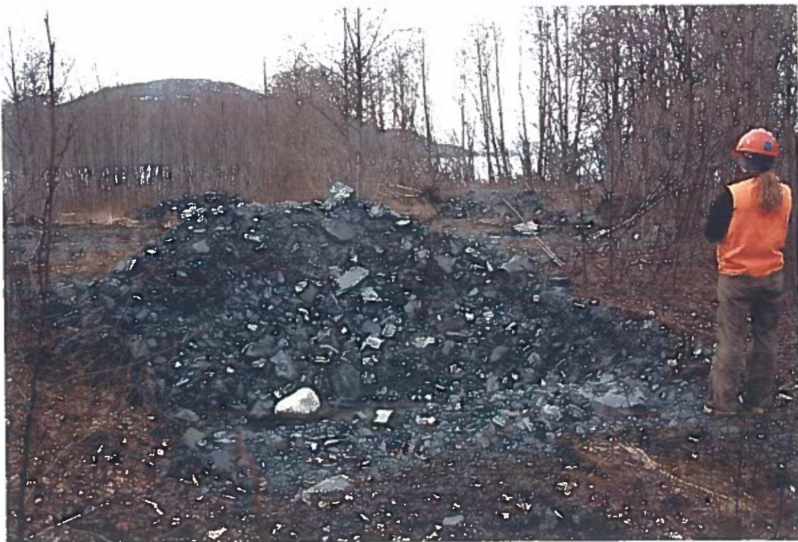
Photo #32: 3/26/12 view looking northwest at one of NORTECH's 10/13/11 exploratory excavations made in the north end of the Mt. Seley storage facility, showing the blue clay & rock making up the 2'-3' thick cap covering the top of the site.
