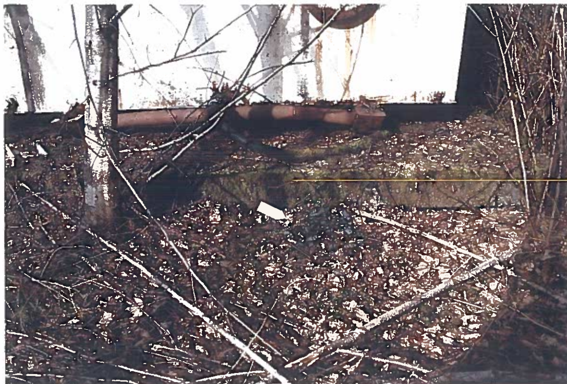
Photo #4: 3/26/12 view of the mill's 20,000-gallon diesel generator tank's east end, where NORTECH's 10/13-14/11 soil sample #GT2 had a DRO level of 1,710 mg/kg.
