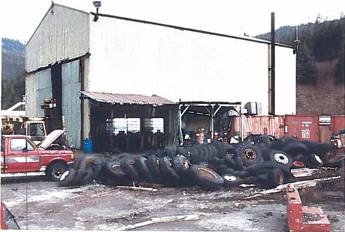
Photo #37: 3/26/12 view looking northwest at the Wrangell Lumber shop's south side, where the lube and hydraulic oil dispensers are located along with a shed for drums, which will be inventoried and evaluated for disposal or recycling as appropriate.
