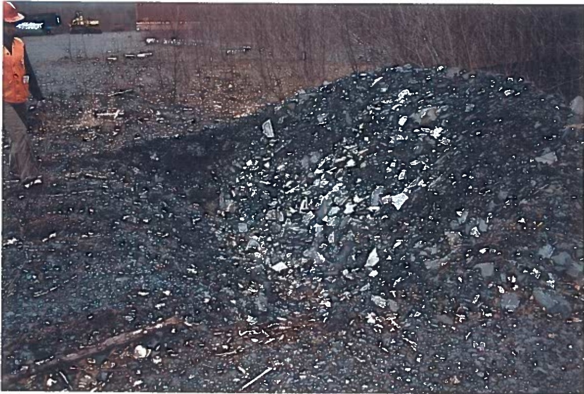
Photo #33: 3/26/12 view looking northeast across the 10/13/12 NORTECH exploratory excavation along the east side of the Mt. Seley storage facility, where sample #TP8 had a slightly elevated DRO level of 302 mg/kg.
