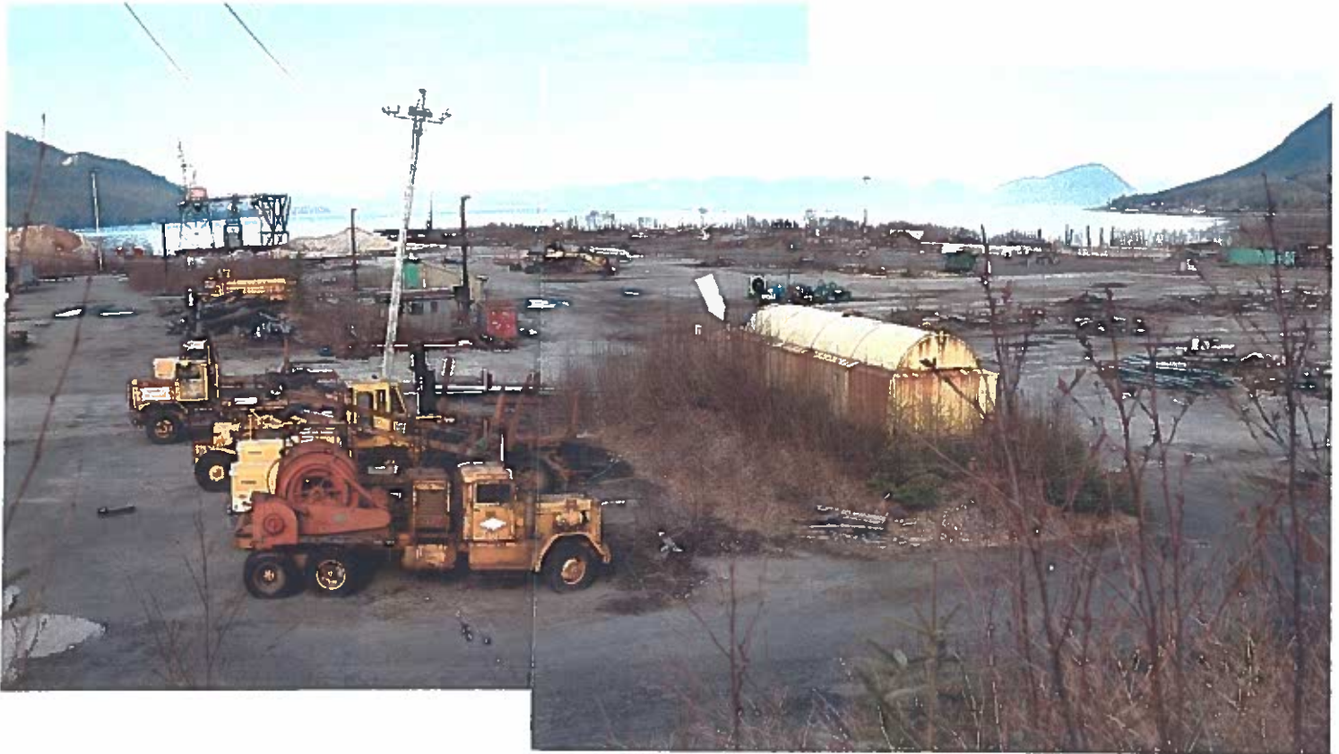
Photo #5: 3/26/12 view looking northwest across Wrangell Lumber's fuel depot, which has a 20,000-gallon diesel oil tank and a 2,000-gallon gasoline tank (arrow) along its west end. See next 3 photos.
