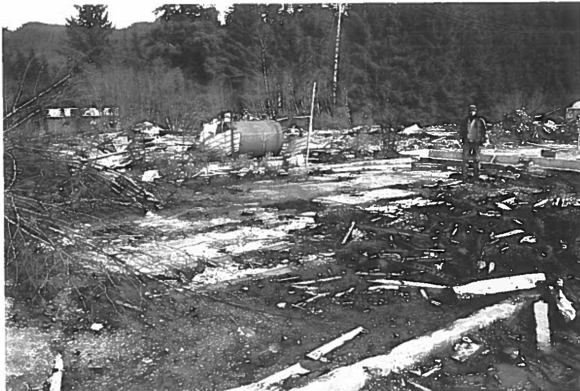
Photo #12: 3/26/12 view looking northeast across the concrete pad for the Wrangell Lumber sawmill building's transformers, showing the former emergency generator concrete pad's 3 empty tanks in the background.
