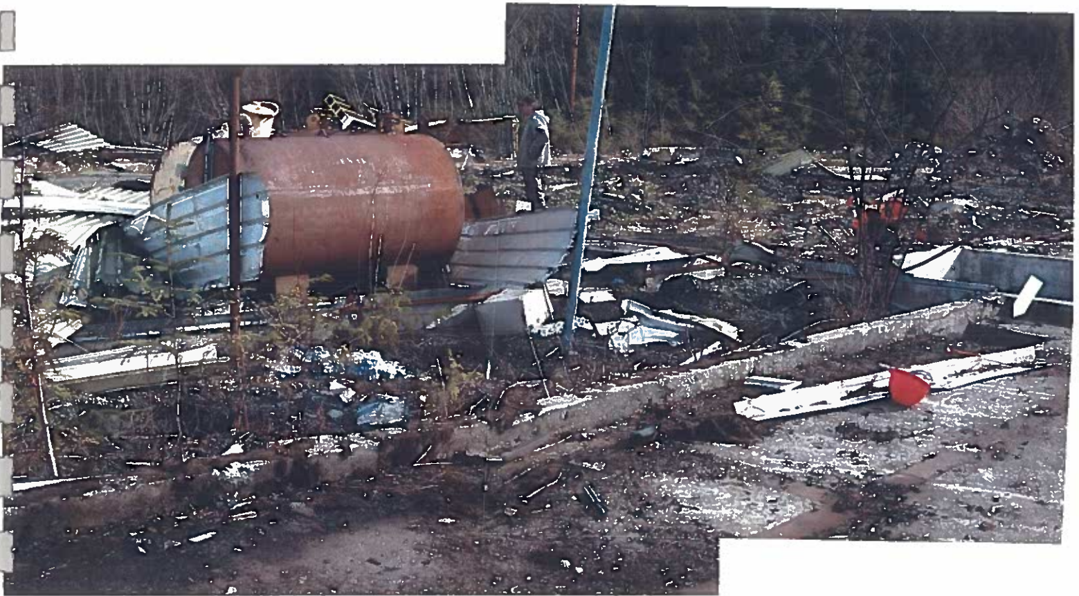
Photo #13: 3/26/12 view looking northeast across the 9'-wide gap between the Wrangell Lumber sawmill's concrete pads for its former transformers (foreground), and the emergency generator building where 3 empty fuel tanks were being stored. Arrow points to the former transformer pad's surface water catchment drain.
