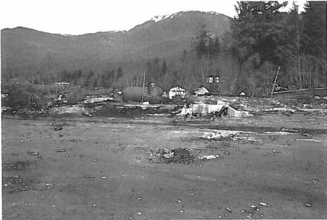
Photo #11: 3/26/12 view looking north-northeast at the 3 empty fuel tanks sitting on the Wrangell Lumber concrete pad for the former emergency generators. See Photos #12 - #20.
