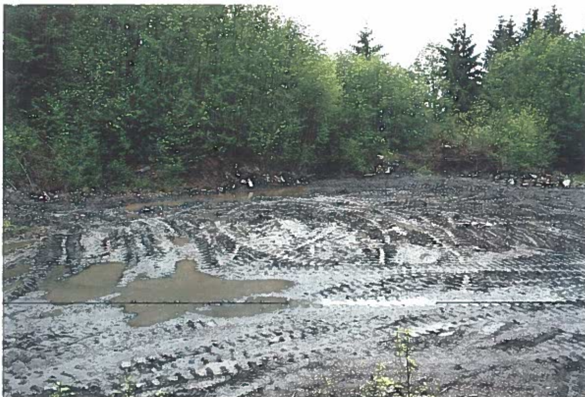
Photo #34: 6/5/12 view looking west across the Wrangell Lumber mill's rock quarry, showing that all of the originally stockpiled contaminated soil had been removed. DRO levels of the two soil samples taken where the 7 loads of soil had been placed were 110-280 mg/kg, and RRO levels were 910-1,400 mg/kg.
