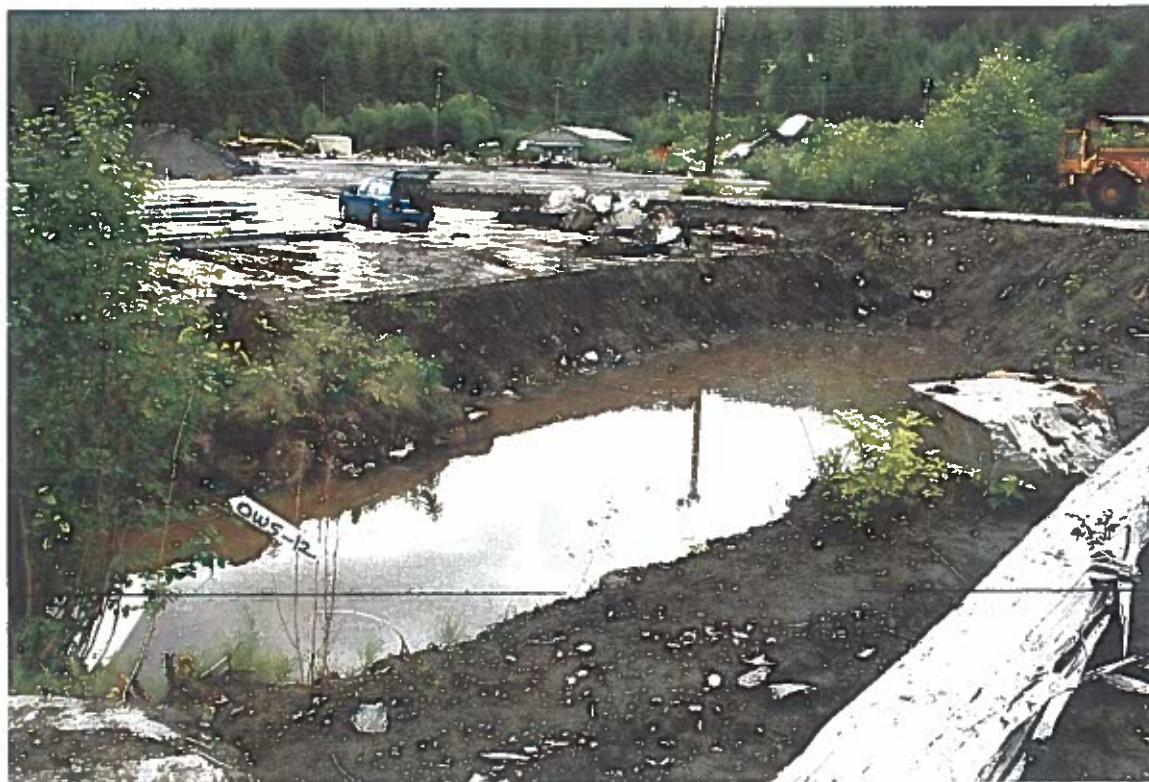
Photo #26: 6/30/12 view looking northeast across the Wrangell Lumber mill site's oil/water separator pond, showing one of the 5 sampling sites along the shoreline of the north side's completed re-excitation.
