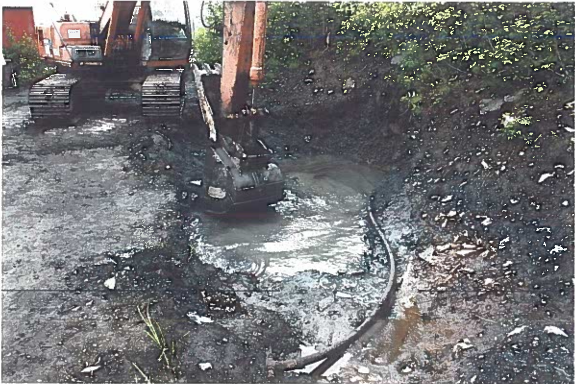
Photo #15: 6/30/12 view of the restarted contaminated soil excavations at the ponded ditchline area behind the Wrangell Lumber mill site's shop building.
