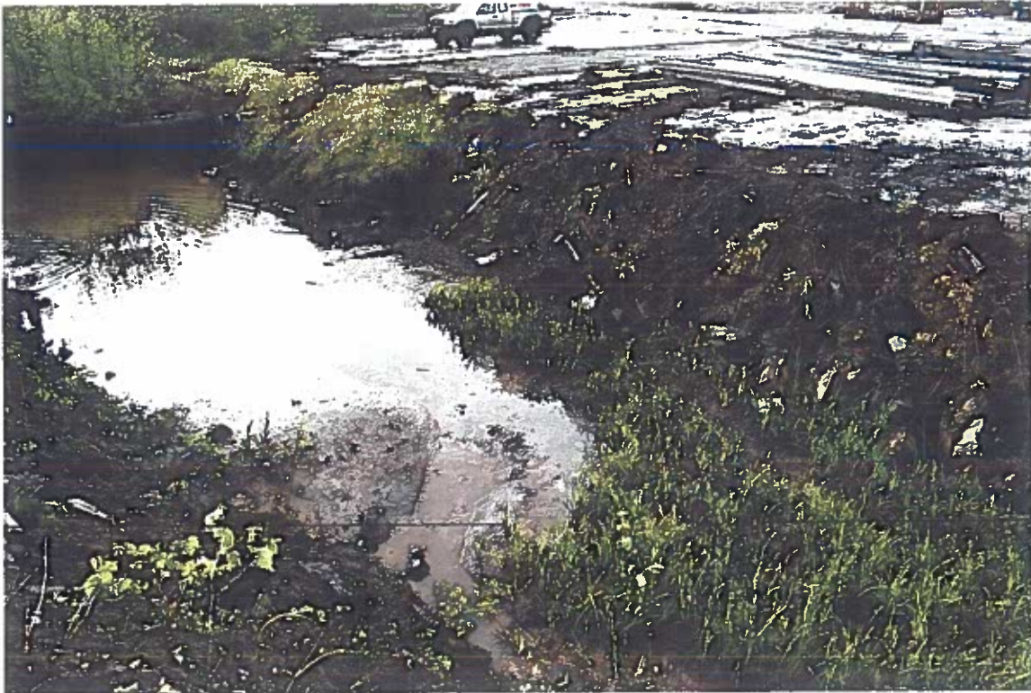
Photo #23: 5/18/12 view looking down on the Wrangell Lumber mill's oil/water separator pond sediment deposits, about to be excavated to a 1'-2' depth. See photo below.
