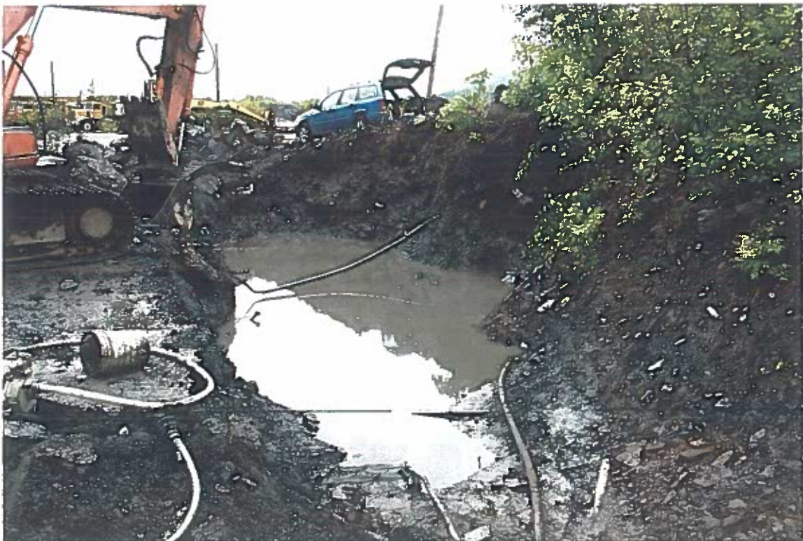
Photo #16: 7/1/12 view of the excavation status of the ditchline ponded area behind the Wrangell Lumber mill shop building, where confirmation sampling was completed along its far northwestern end. Contaminated soil still remains along the pond's lower portion, and likely extends a foot or more beneath the asphalt pavement.
