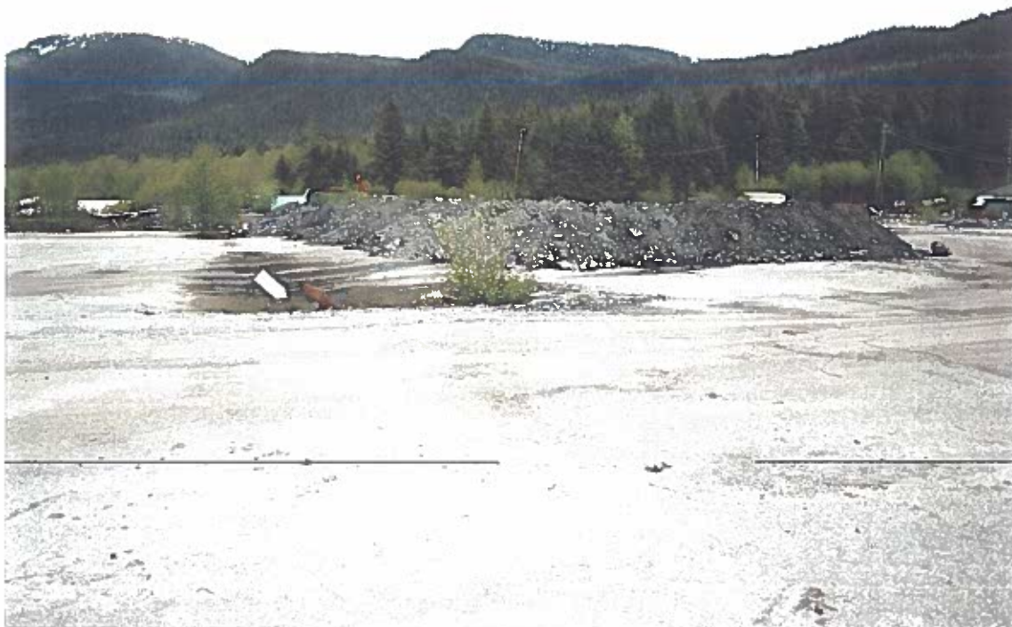
Photo #31: 5/19/12 view of the initial contaminated soil stockpile on the Wrangell Lumber mill's concreted area. Arrow points to a roadway culvert inlet, one of several that drained the area to the oil/water separator pond.
