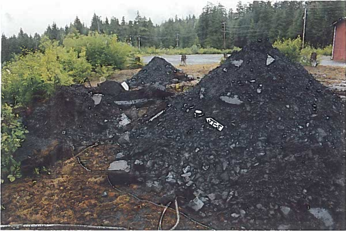
Photo #1: 7/1/12 view looking north across the three piles of excavated soil from the Wrangell Lumber mill site's Jet-A Tank cleanup site, showing two of the 5 samples to confirm whether ADEC cleanup criteria have been met. The unmarked arrow shows the 4.5'-deep excavation site, see photo below.
