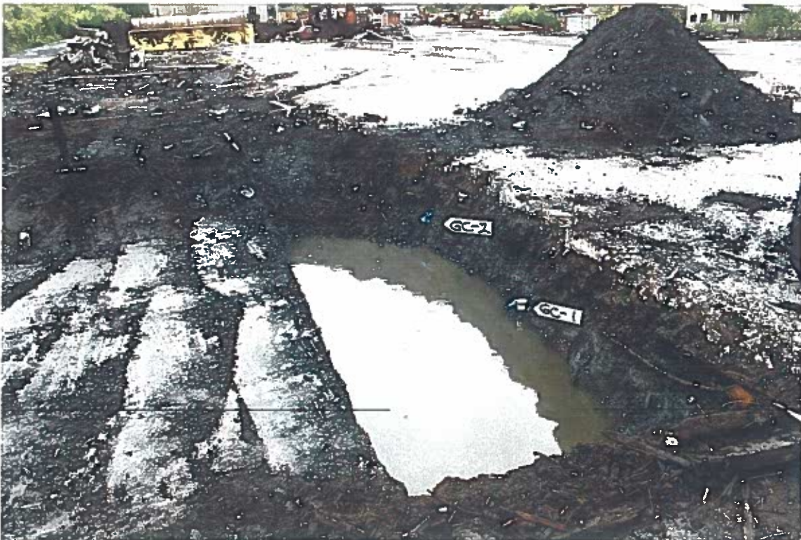
Photo #28: 6/5/12 view looking southwest across the 2'-deep exploratory excavation at the north end of the Wrangell Lumber mill's former green chain area. Sample GC1 had DRO/RRO levels of 5,500 & 15,000 mg/kg, and GC-2's levels were 11,000 & 25,000 mg/kg.
