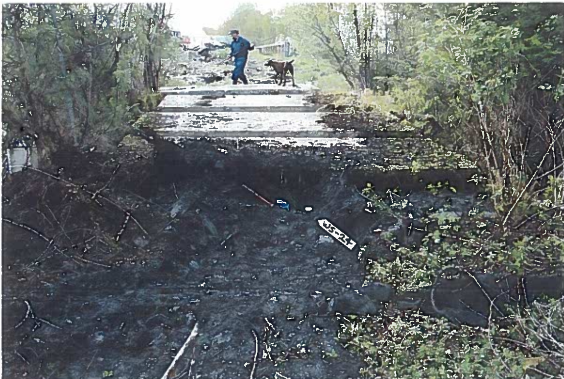
Photo #4: 5/17/12 view looking west across the Wrangell Lumber mill's electric generator tank site excavation. No soil was removed & the two confirmation samples easily met cleanup criteria (DRO = 160-180 mg/kg, RRO = 220-440 mg/kg).
