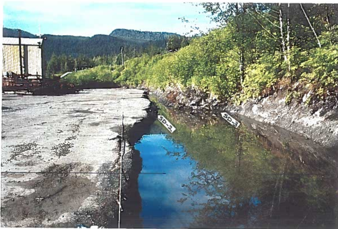
Photo #13: 6/4/12 view of the Wrangell Lumber mill site's shop drainage ditch and sump, now cleaned with vegetation removed. The sampling control line started from the former sump outlet, and crossed the shop ditchline 260' away where it turned behind the shop building.
