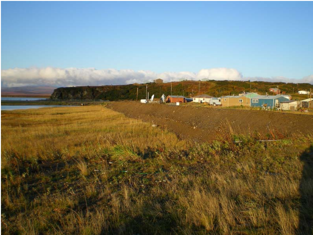
Figure C7. Berm protecting infrastructure of lower town area.
