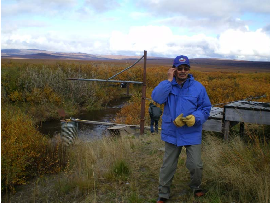
Figure C4. Looking northeast at drinking water intake. Toby Anungazuk in foreground.
