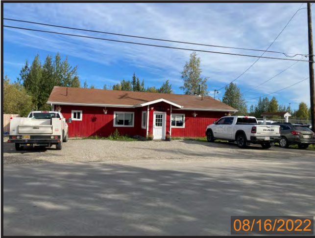
PHOTOGRAPH 1: VIEWED NORTH- SUBJECT PROPERTY- SOUTH SIDE
