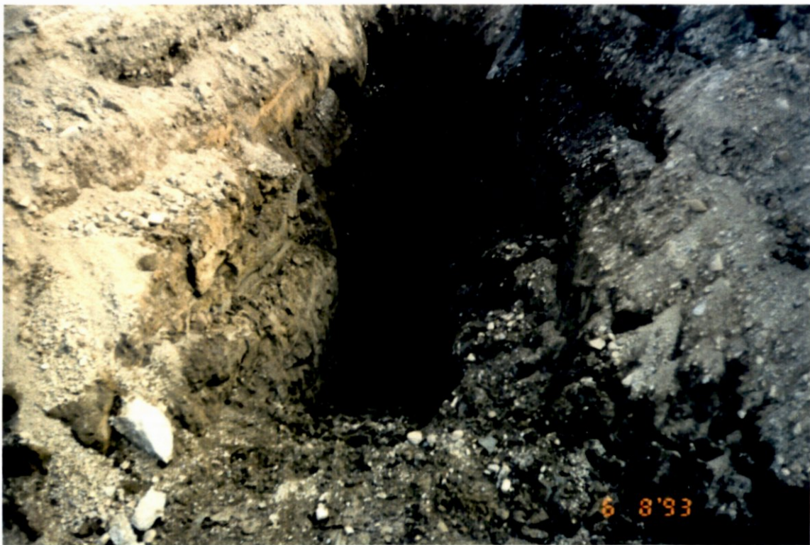
Photograph 4 - Excavating to determine vertical limits of contamination.
