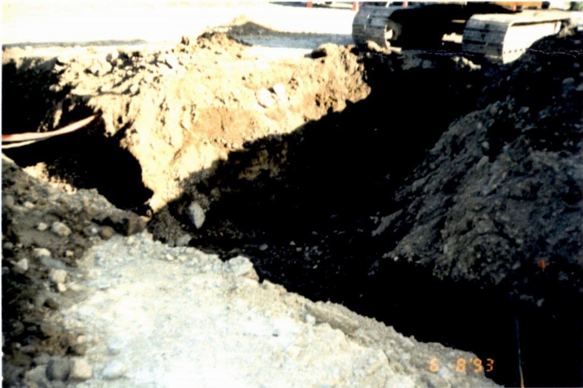
Photograph 3 - Excavating perpendicular to drainpipe to determine horizontal limits of contamination.
