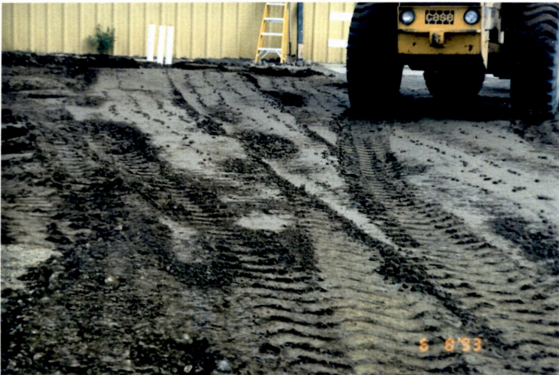
Photograph 6 - Work area at completion of site activities.
