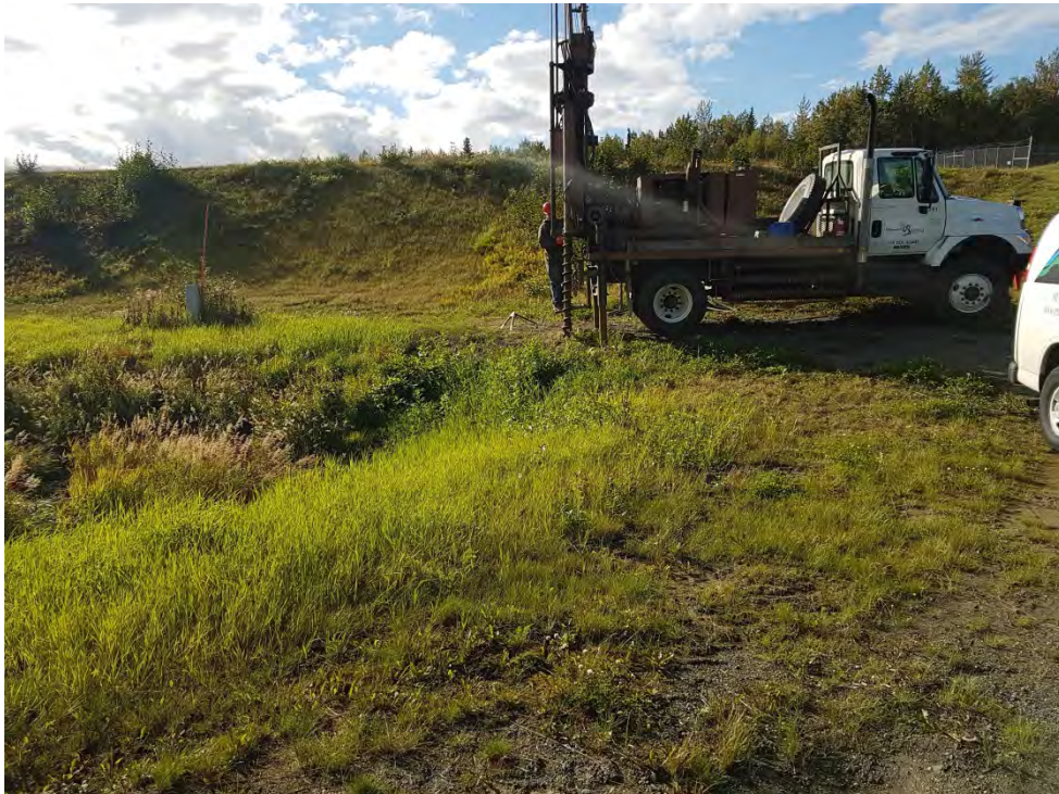
Photo 2: View of monitoring well site, looking east.
