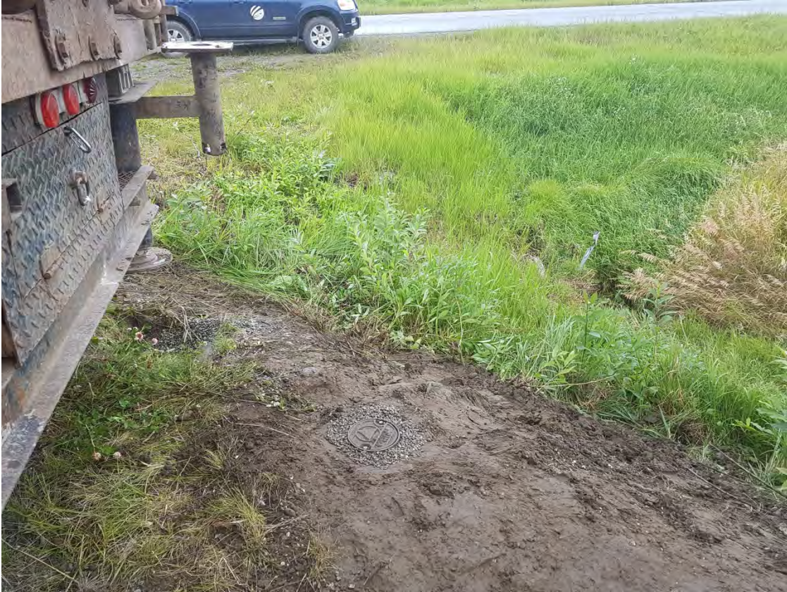
Photo 3: View of Monitoring Well MW-04 flush mount after installation.
