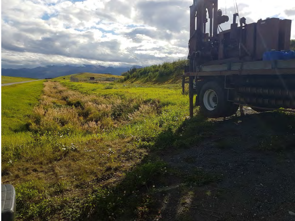
Photo 1: Monitoring Well MW-04 installation site, looking south.
