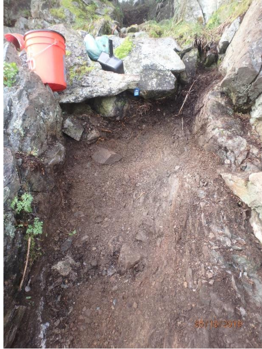
Photograph 7: May 10, 2019 Weathered friable bedrock below removed soil
