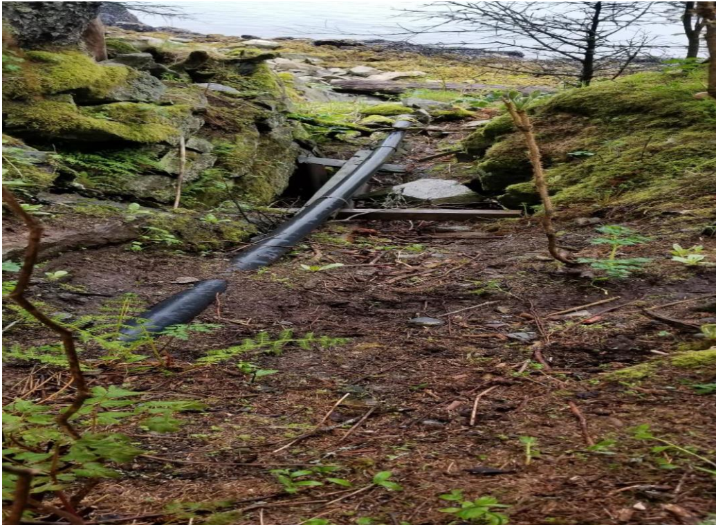
Photograph 5: May 10, 2019 Outfall pipe terminating above the high tide line
