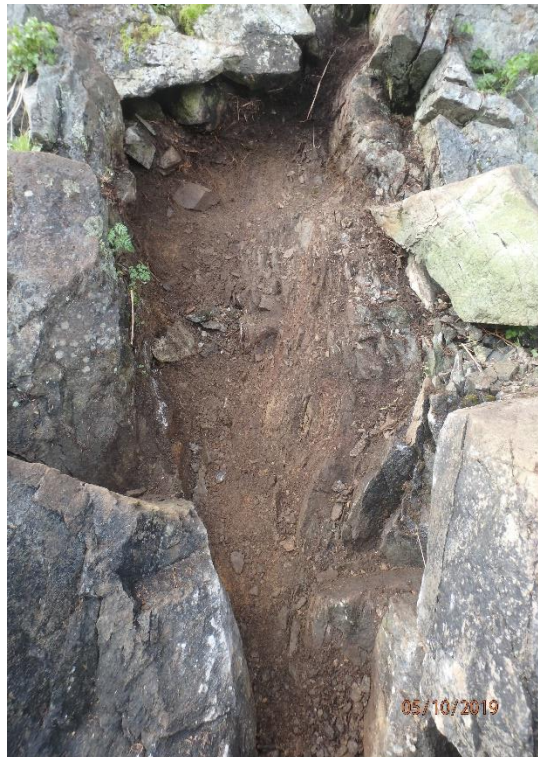
Photograph 8: May 10, 2019 All soil removed down to bedrock
