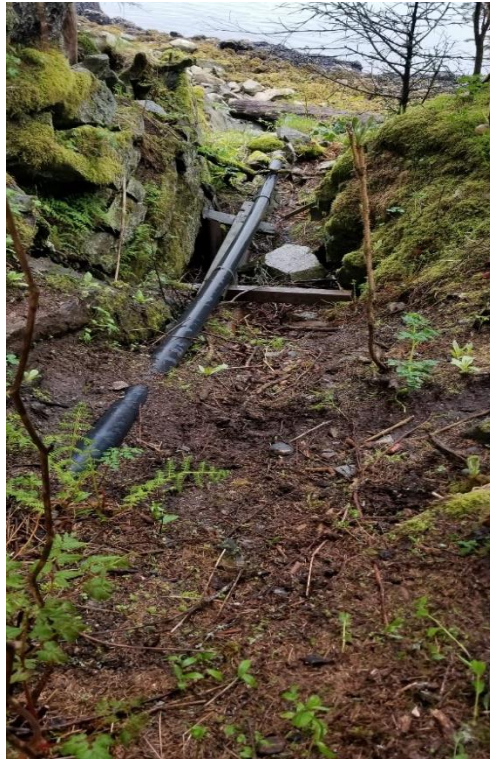
Photograph 3: May 10, 2019 Assay lab outfall discharge pipe
