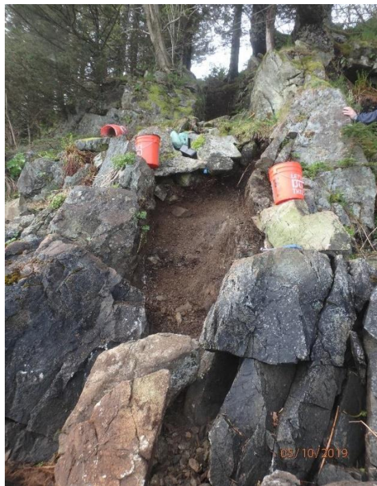
Photograph 6: May 10, 2019 Soil removal at discharge zone of removed pipe
