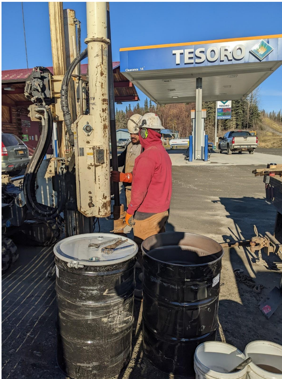
Photo 1: Looking north, Discovery advancing Boring B5 (October 24, 2022)
