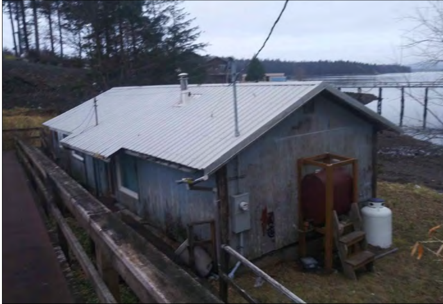
PHOTO 1 Active HOT and Propane Tank.
