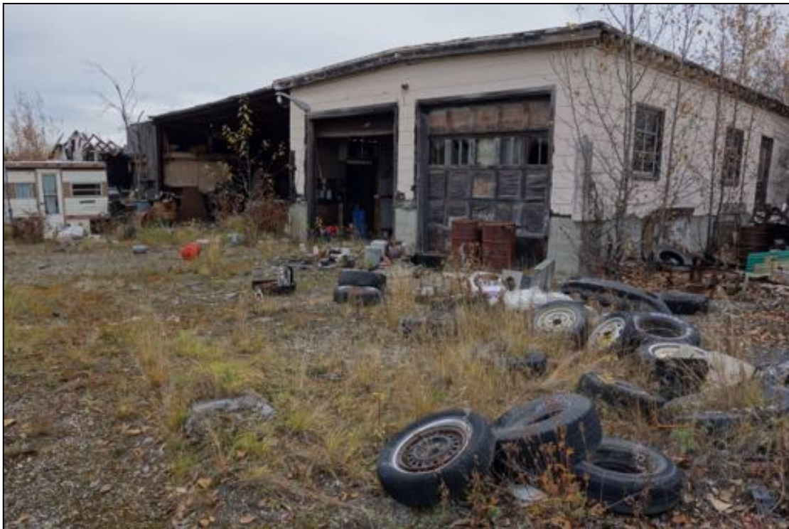
PHOTOGRAPH 30: TWO BAY SHOP LOCATED IN WESTERN PORTION OF SITE; LOOKING NORTHEAST. 9/22/16.
