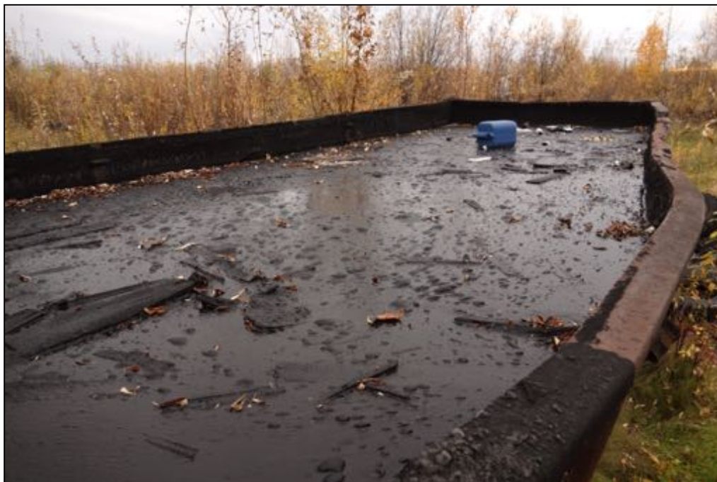
PHOTOGRAPH 4: RAIL CAR FILLED WITH TAR (SEE FIGURE - AREA OF INTEREST #2); LOOKING SOUTHEAST. 9/22/2016.
