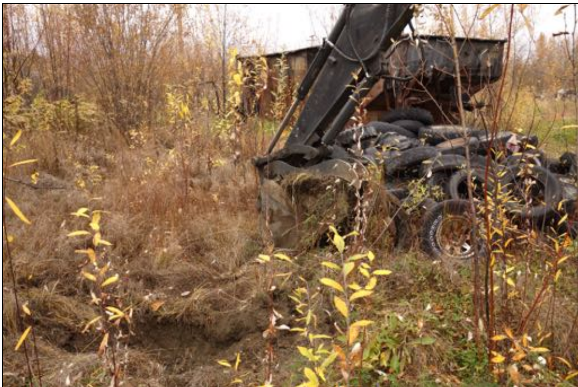
PHOTOGRAPH 6: DIGGING TEST PIT (TP-6) NEAR POOLED TAR; LOOKING NORTHWEST. 9/22/2016.
