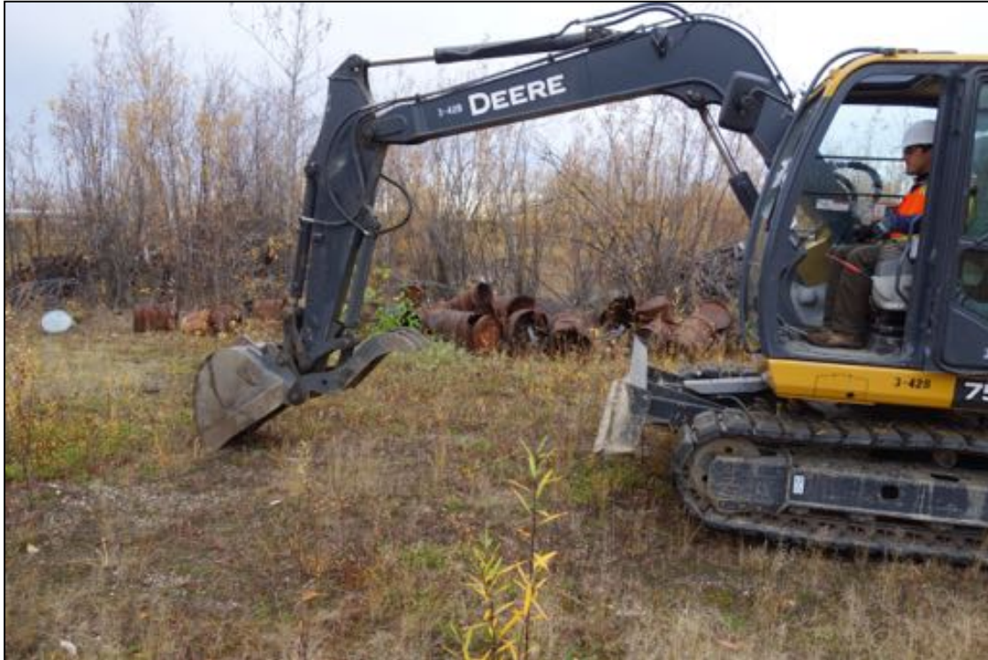
PHOTOGRAPH 7: DIGGING TEST PIT (TP-8); LOOKING SOUTH. 9/22/2016.
