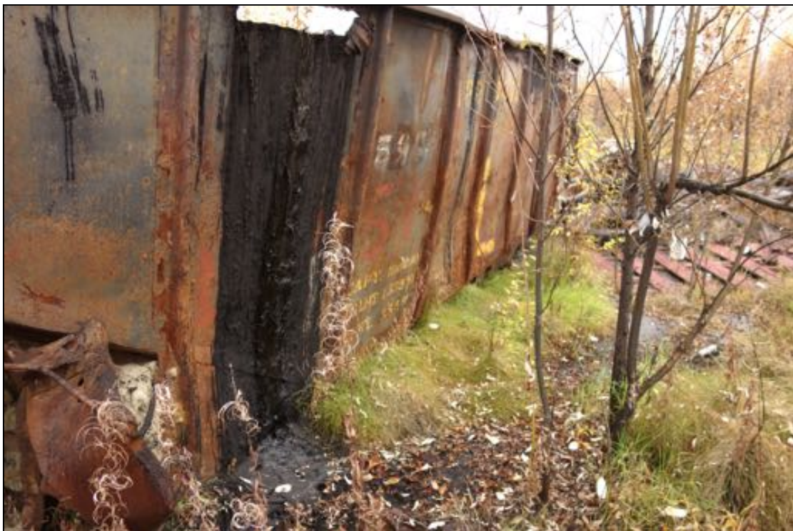
PHOTOGRAPH 2: RAIL CAR WITH TAR ON NORTHWEST PORTION OF PROPERTY (SEE FIGURE - AREA OF INTEREST #2); LOOKING SOUTHEAST. 9/22/2016.
