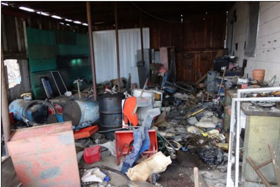
PHOTOGRAPH 32: NORTHERN HALF OF SHOP; DRUMS WITH UNKNOWN CONTENTS OBSERVED; OIL STAINING ON FLOOR; LOOKING WEST. 9/22/16.
