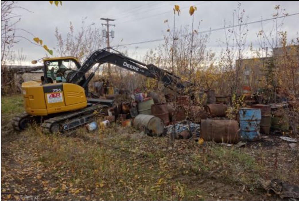
PHOTOGRAPH 33: AREA WITH APPROX 40 DRUMS WITH UNKNOWN CONTENTS (POSSIBLY GAS AND/OR WASTE OIL); OIL STAINING OBSERVED ON GROUND (SEE FIGURE – AREA OF INTEREST #1); LOOKING SOUTHWEST. 9/22/16.
