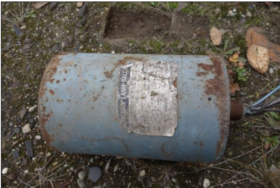
PHOTOGRAPH 28: MERCURY LIGHT BALLAST (M-1) LOCATED WEST OF THE ONSITE SHOP. 9/22/16.
