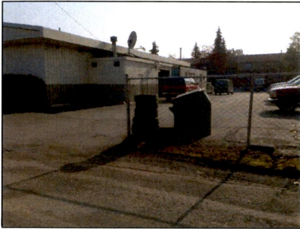
1. View of the rear of the Site facing east
