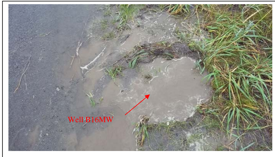
Photo 1: Monitoring Well B16MW is flooded with surface water from overnight rainfall (August 19, 2011).
