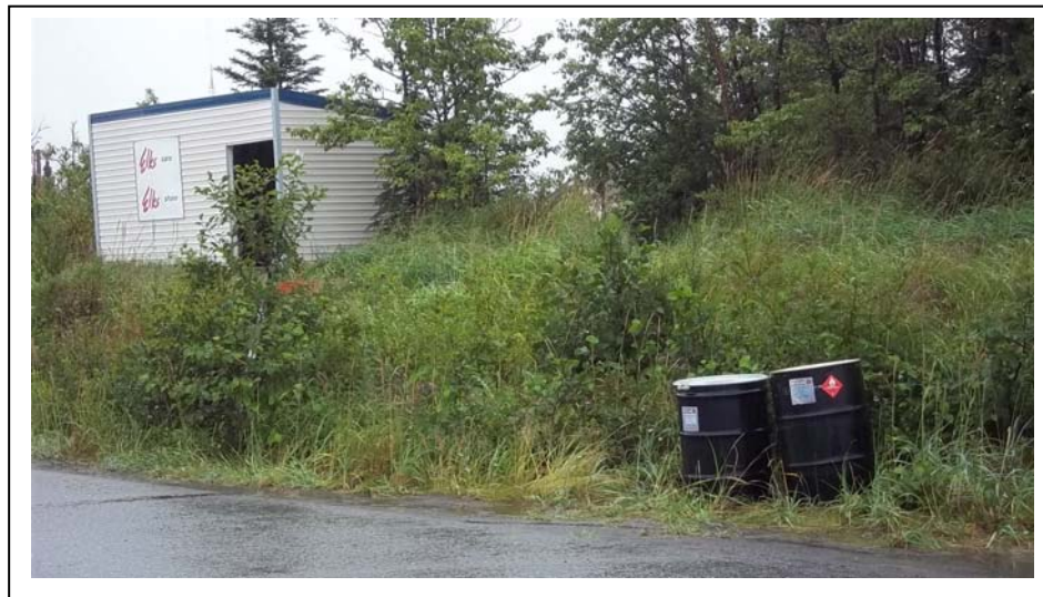
Photo 2: 55-gallon drums containing purgewater and product removed from monitoring wells, prior to transport for disposal (August 19, 2011).
