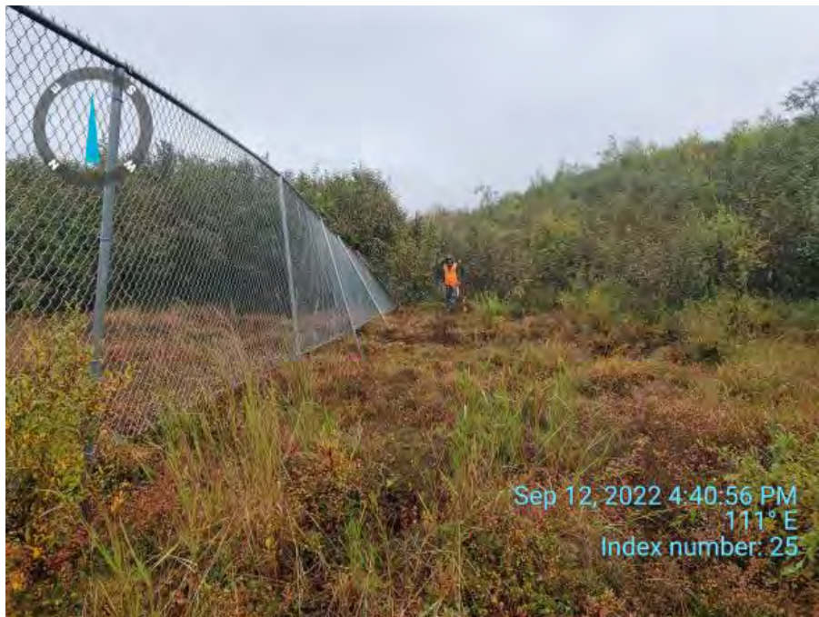
Photo ID: Index 25. View southeast. Eastern exclusion fence with post frost-jacked and leaning at 45-degree angle. Alders entwined in fence.
