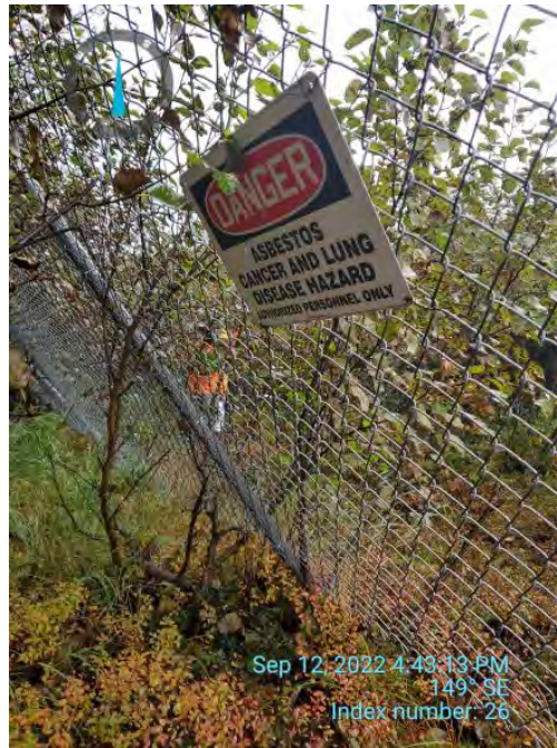
Photo ID: Index 26. View southeast. Asbestos warning sign hung on eastern exclusion fence. Fence leaning at 45-degree angle.
