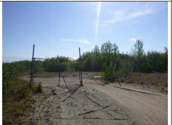
PHOTO 4: Southern gate has been extensively vandalized to allow for trespassing by vehicles. Note signage present on ground, but otherwise in good condition.
