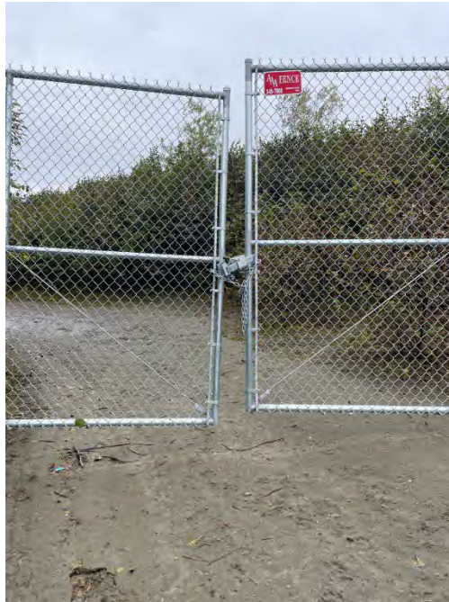
Photo ID: BE002. View south. Northern gate secured with locked chain. Prevents vehicles/ATVs access but not trespassers on foot.
