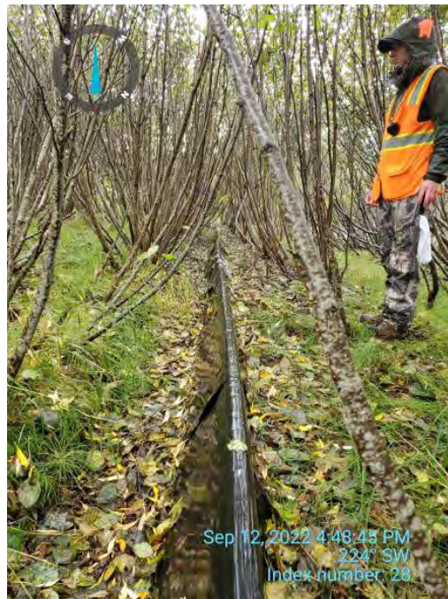
Photo ID: Index 28. View southwest. Lined drainage channel within eastern exclusion fence area, in good condition. Photo shows dense, tall alder growth characteristic of eastern and western cap areas.
