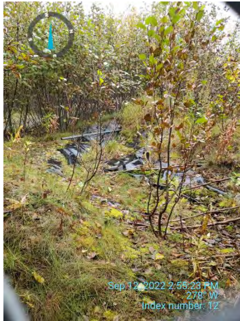
Photo ID: Index 12. View west. Lined drainage channel within exclusion fence at south corner adjacent to ATV trail. No sign of breaching contributing to ATV trail erosion.
