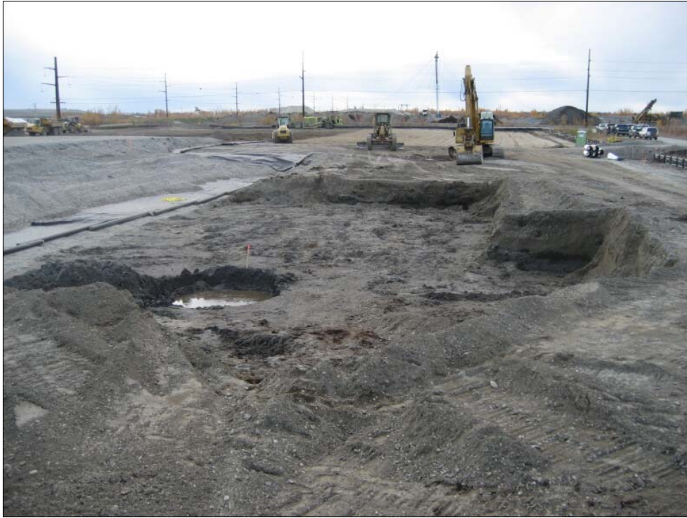
Photo 9 - Final limits of corrective action excavation looking south 9-26-08, exploratory pit to groundwater at left
