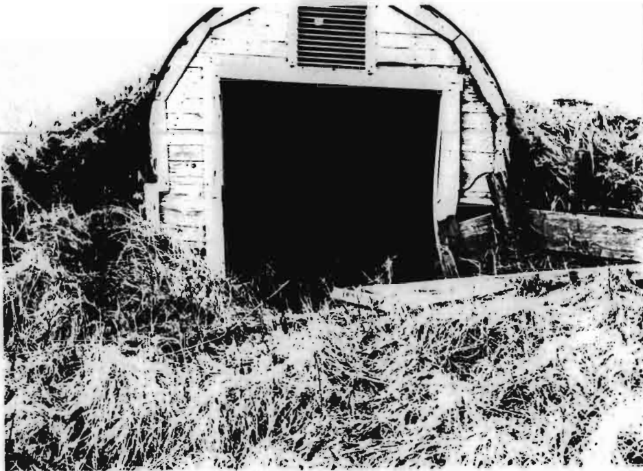
Power plant shelter - Elephant steel 10' x 15' Ugadaga Bay
