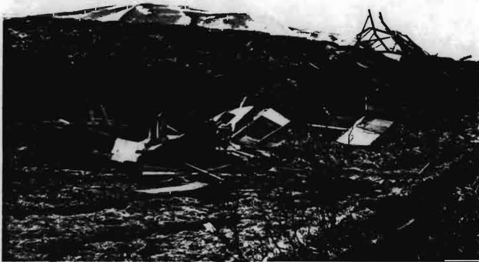
Latrine and Utilities - Quonset Hut - Ugadaga Bay
