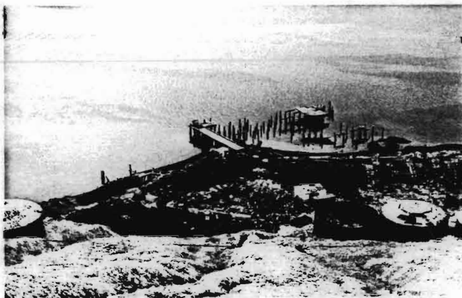
Whaling station on Akutan Island old and new dock, crab pot storage and old fuel oil storage tanks - Akutan Island
