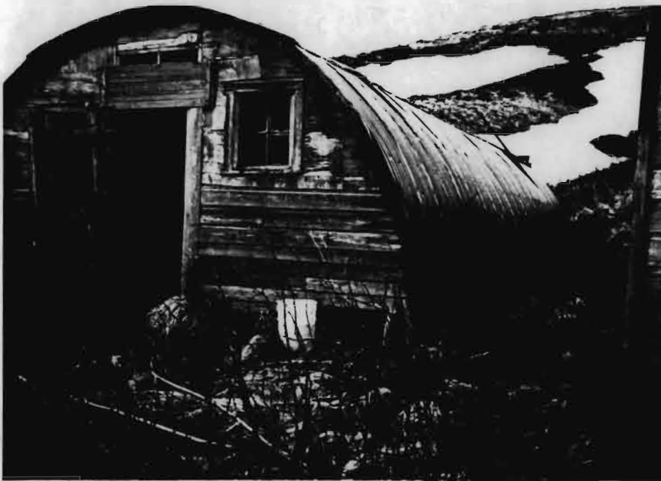
Quonset Hut 10' x 32' - Eider Point
