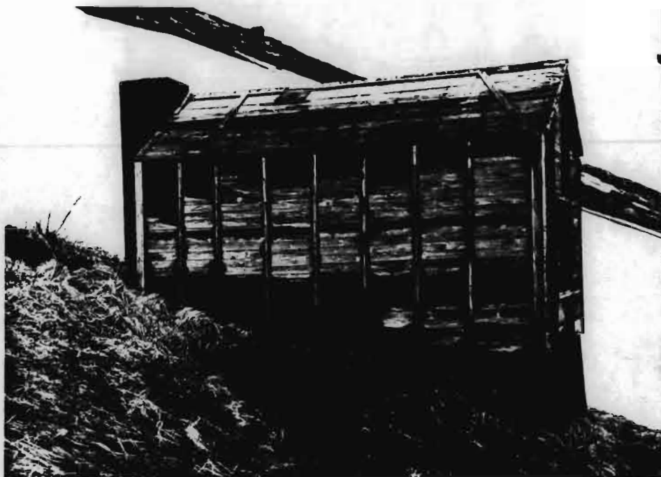
Incinerator building - concrete and wood - Eider Point
