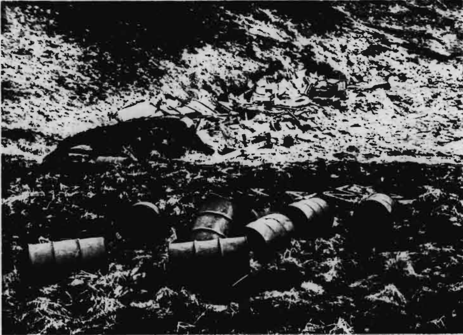
Barrels, Power plant shelter - Elephant steel 10' x 15' and collapsed barracks (Pacific Huts) - Ugadaga Bay
