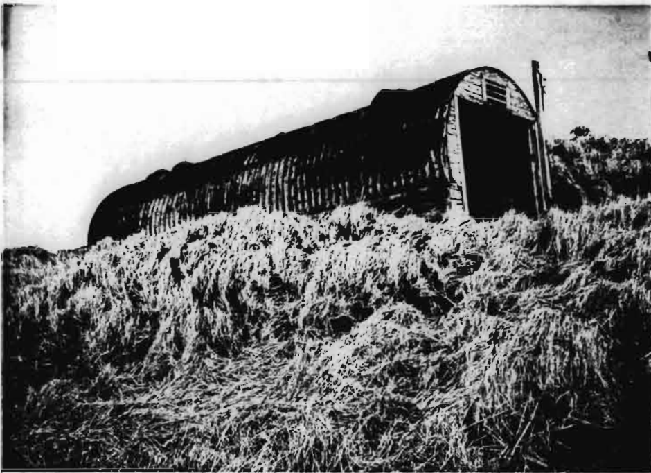
Searchlight shelter - Erskine Point
