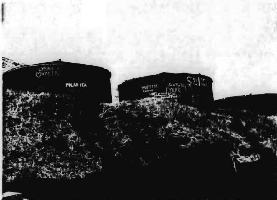
Fuel oil storage tanks - Akutan Island
