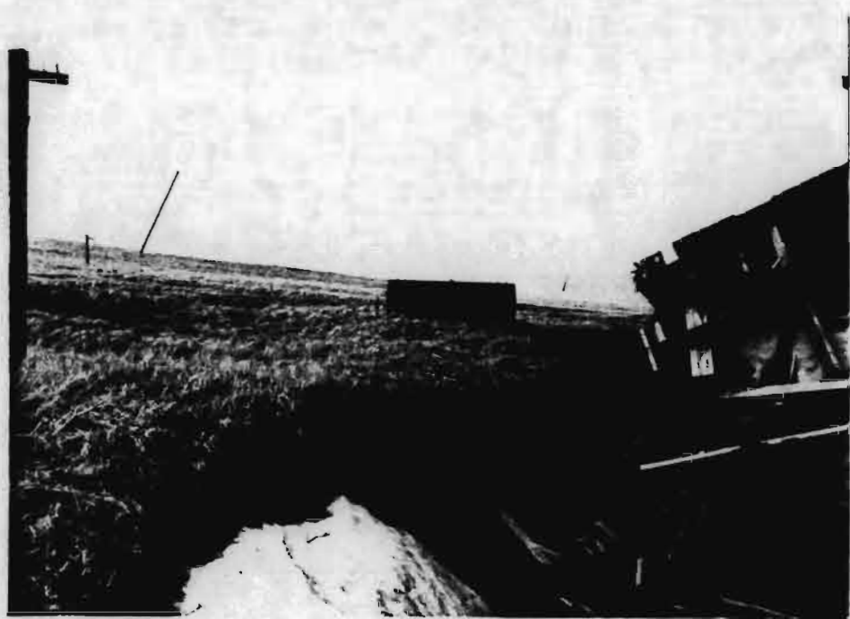
1000 gallon tank - Cape Wislow
