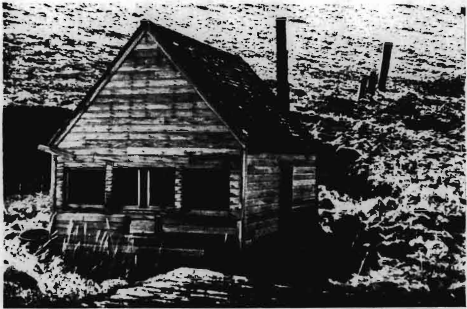
Tram winch shelter - Cape Wislow
