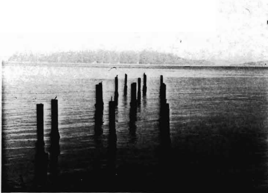
Remaining piles old dock - Eider Point
