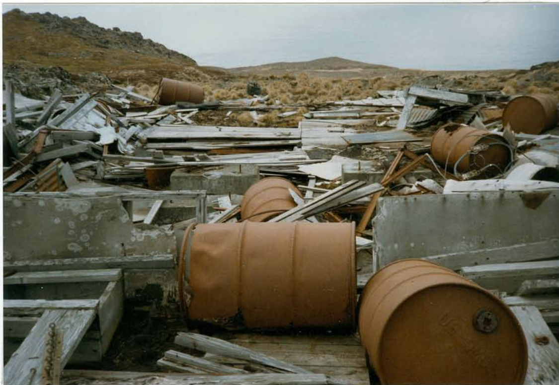
REMAINS OF GENERATOR BUILDING
