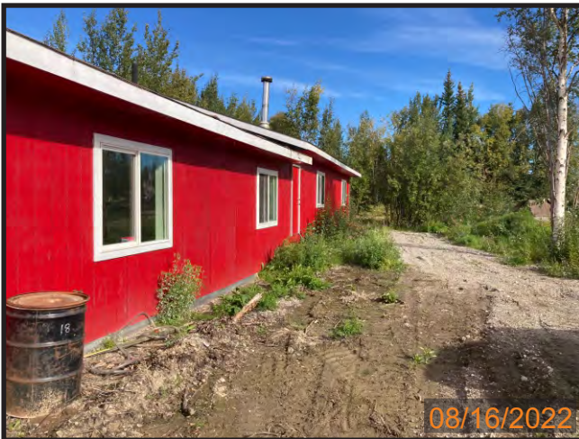
PHOTOGRAPH 3: VIEWED NORTH- SUBJECT PROPERTY EAST SIDE- BOILER ACCESS DOOR IN MIDDLE
