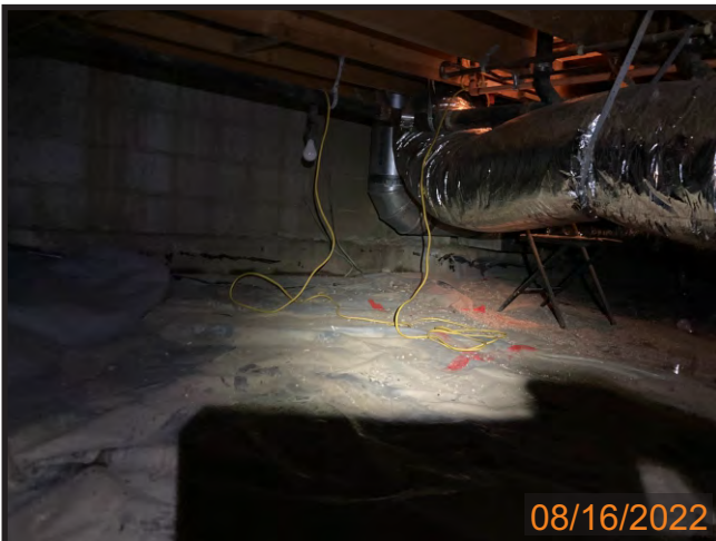
PHOTOGRAPH 5: VIEWED SOUTHEAST- CRAWL SPACE BELOW ACCESS HATCH
