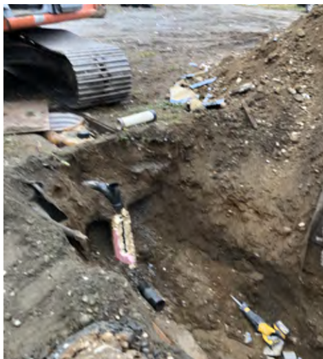
Photo 5: Excavation sidewall near septic.
