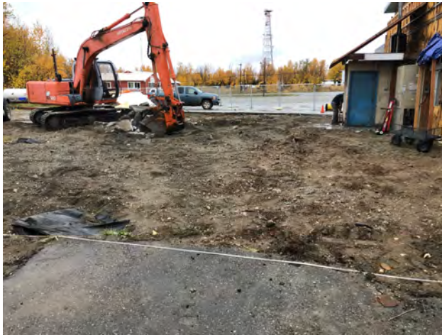
Photo 1: Contractor clearing remaining slab rubble.
