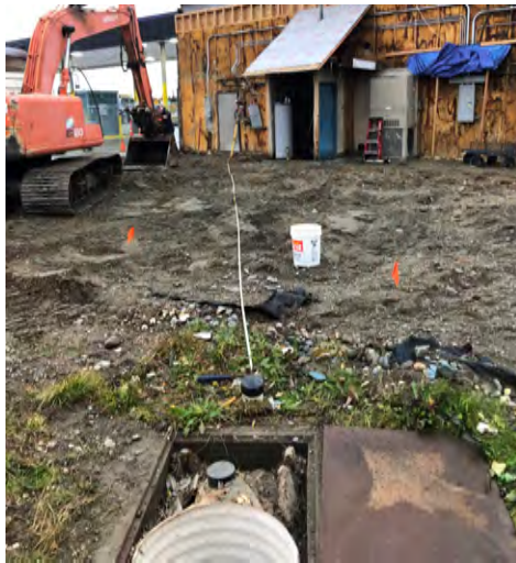
Photo 3: Measuring distance from septic to building.
