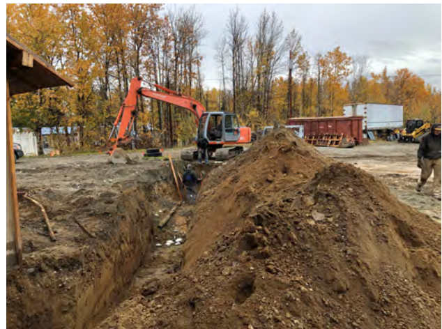
Photo 4: Excavation from building to septic with side-cast soils.
