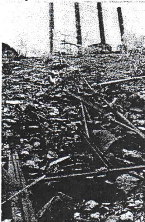
Debris Pile below Power Plant
