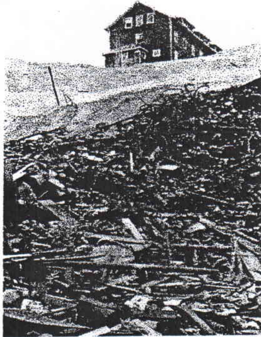
Debris pile below West Bunk house
