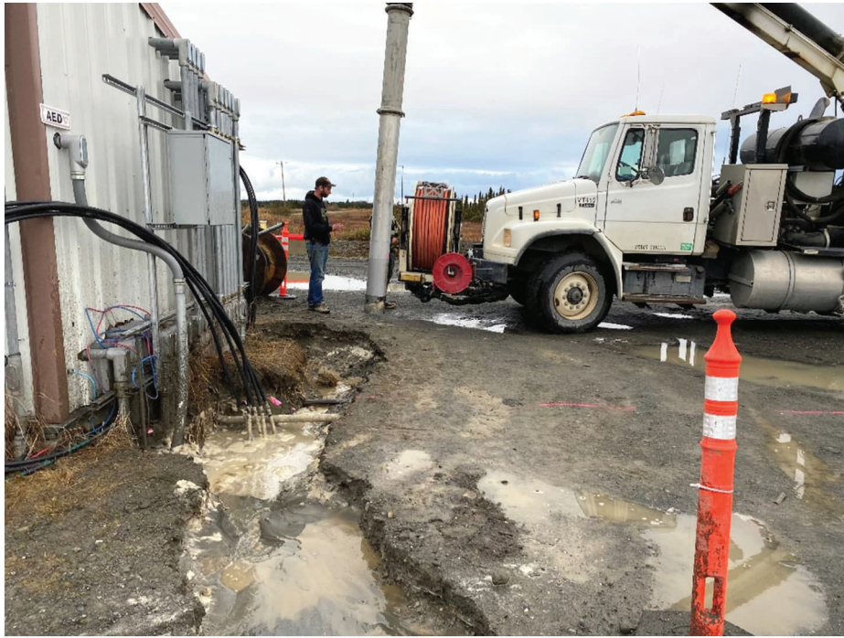
Photo 7: View of water dewatering activities. Photo taken facing south (October 13, 2023).
