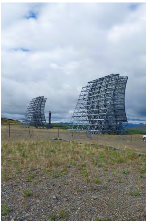
Photograph 2: Antennas on east side of former installation, view north.
