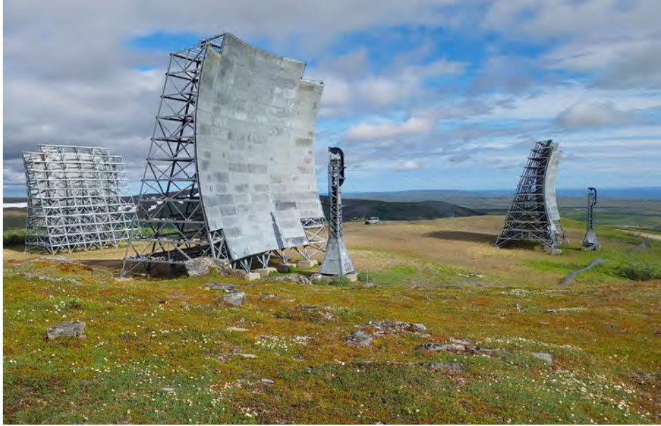
Photograph 7: Overview of former installation area and antennas, view southeast.
