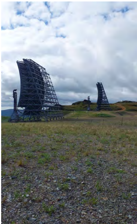
Photograph 1: Southern antennas, view west.
