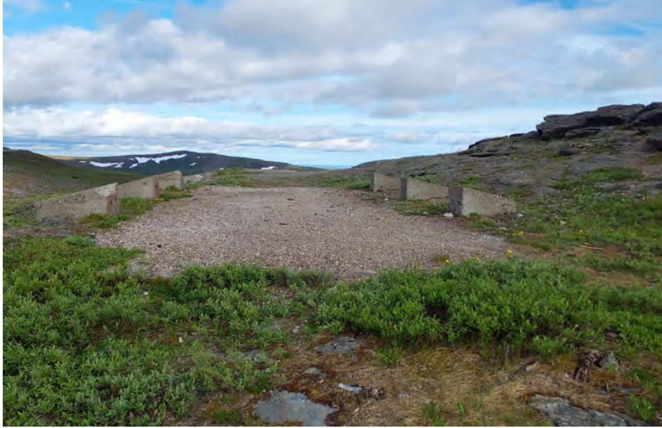
Photograph 13: Unknown former foundation, view southeast.
