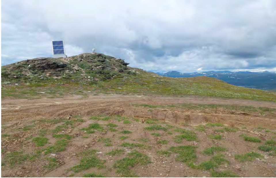
Photograph 9: Solar panel and monitoring equipment, view north.
