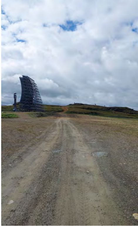
Photograph 3: Northwest antenna and former infrastructure location, view north.
