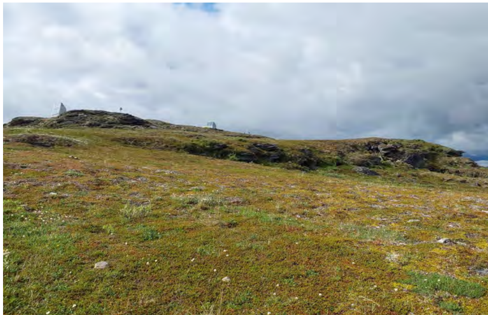
Photograph 4: Solar panels and monitoring equipment, north of former installation, view north.
