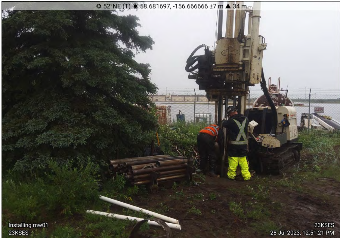
Photo 2. Installing MW-01, looking North. Date: 7/28/2023.
