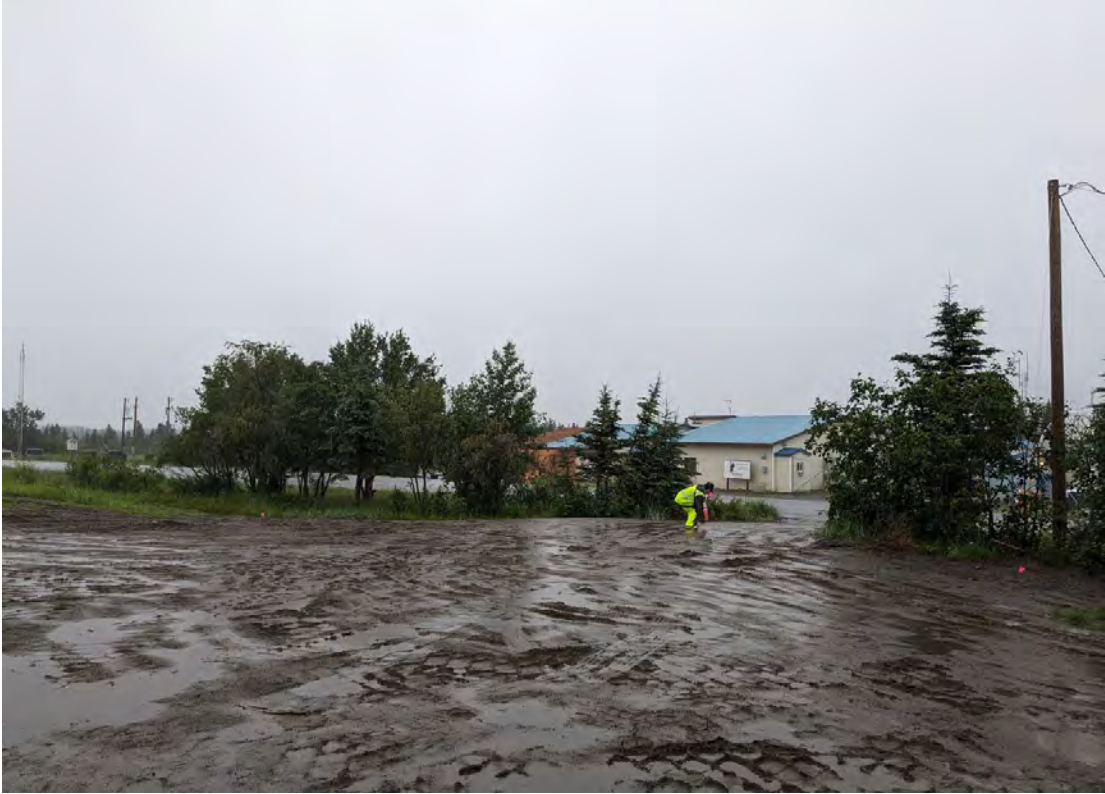
Photo 1. Overall site, looking south. Date 7/28/2023
