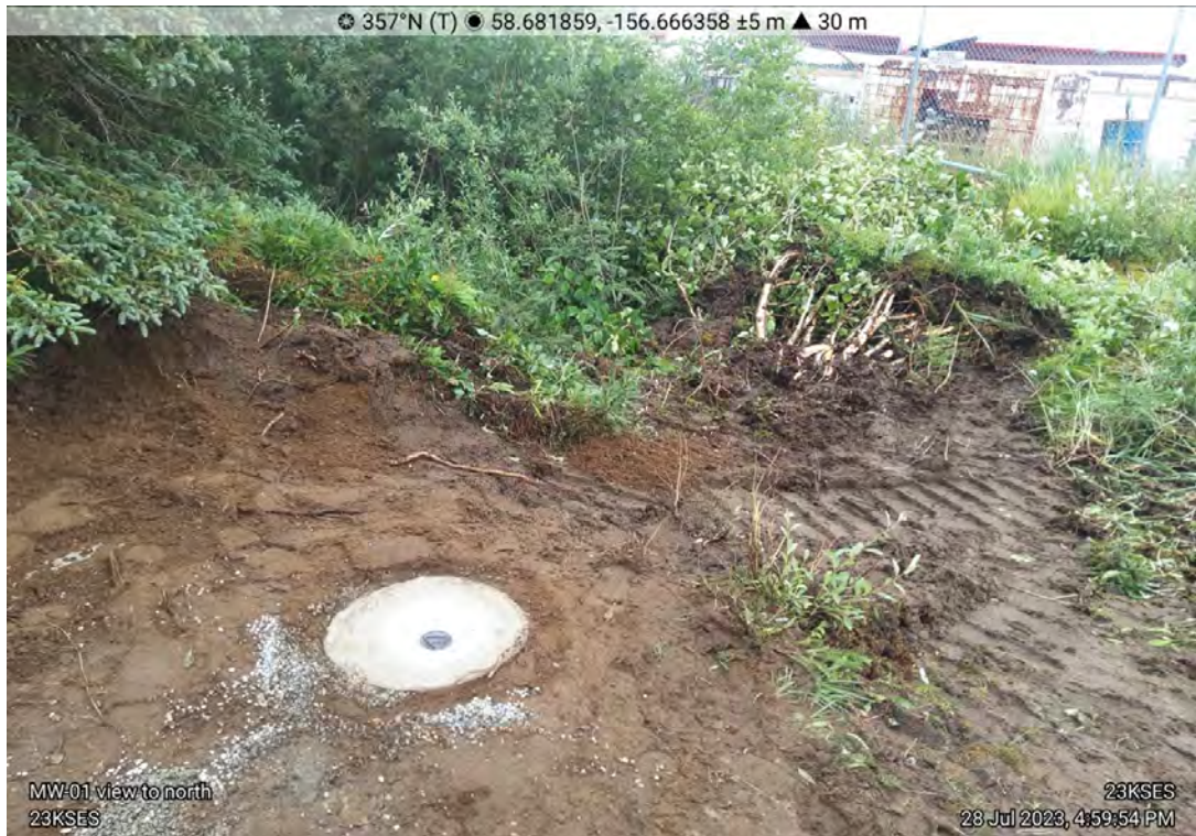
Photo 3. MW-01 installed, looking North. Date: 7/28/2023
