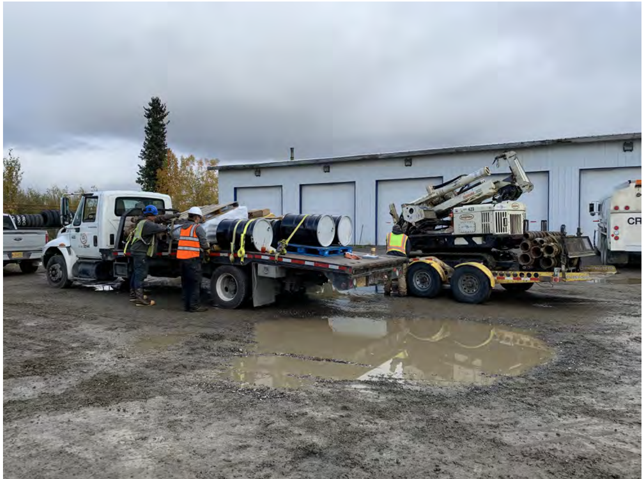
Photo 7: Drillers preparing the drill rig.
