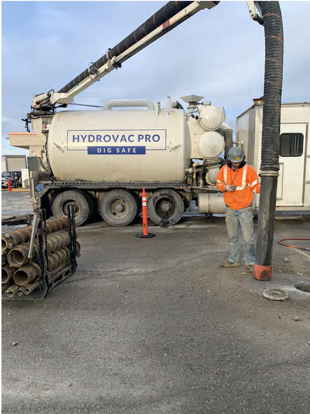
Photo 8: HydroVAC Pro vacuuming the gravel fill from the drill area.
