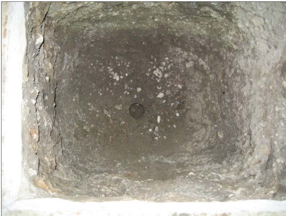
Photo 04 - Bottom sampling location (typical)
