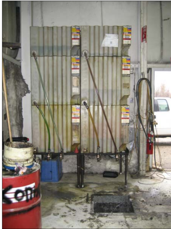
Photo 03 - FD-05 after removal of the structure and prior to sealing
