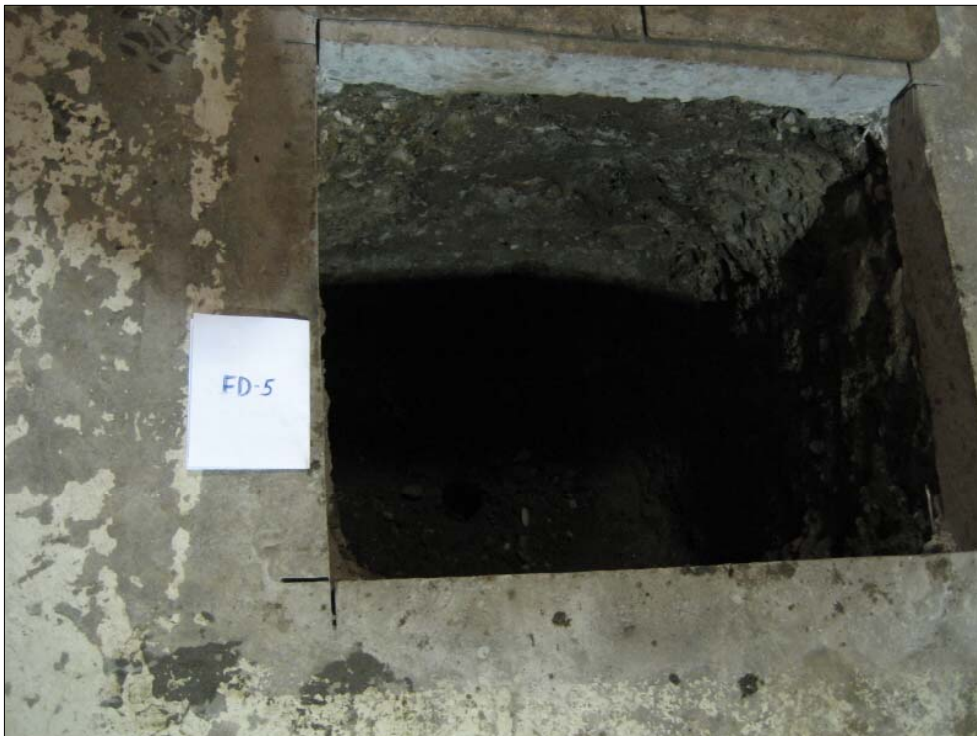
Photo 02 - FD-02 after removal of the structure and prior to sealing
