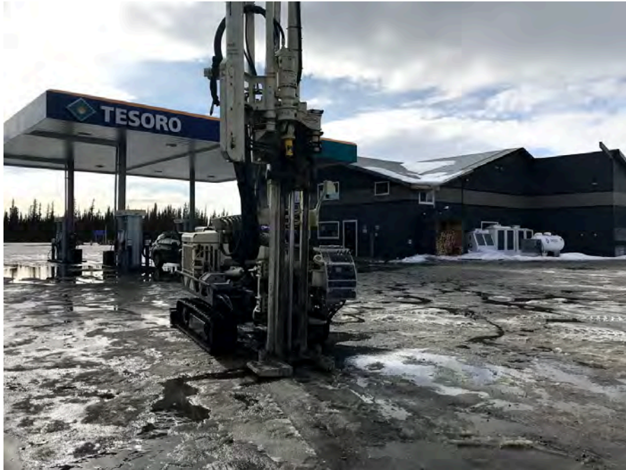
Photo 1: Drilling Boring B1 near the source area, facing west. (April 12, 2021)
