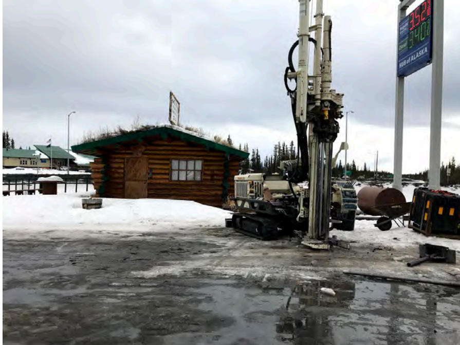
Photo 3: Drilling Boring B7 east of source area, facing east. (April 13, 2021)
