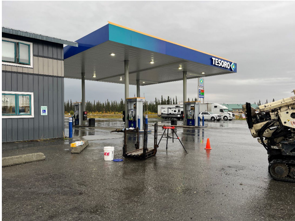
Photo 5: Soil Borings. B17 to the west of source area. (September 13, 2022)
