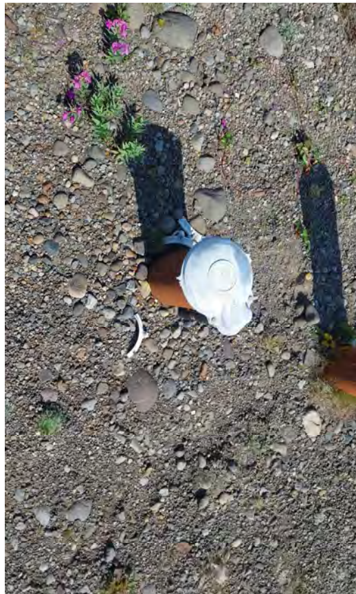
Photograph 12: Installation drinking water wellhead. View oblique.
