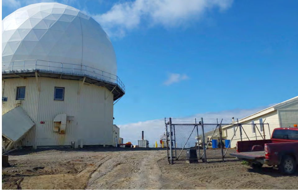
Photograph 1: Front gate with radar dome and module living train. View west.
