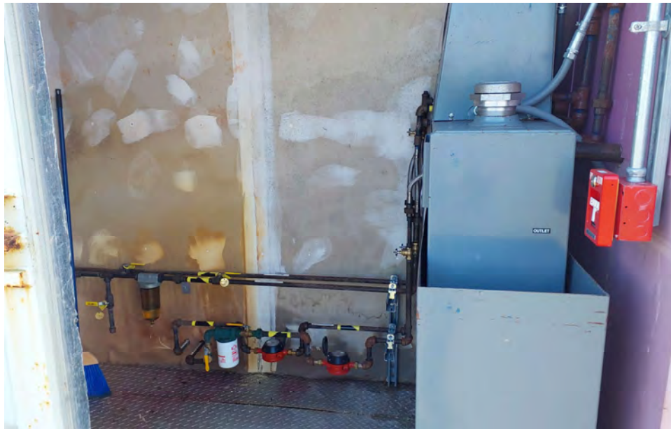
Photograph 6: Non-operational incinerator shed diesel day tank. View oblique.
