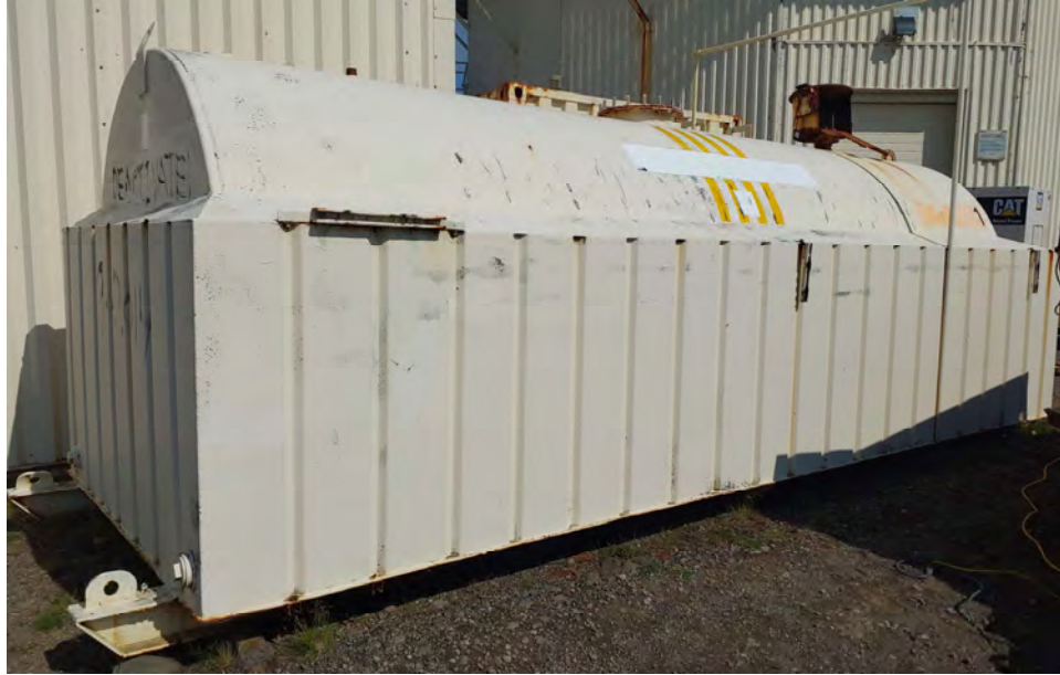
Photograph 9: Bulk diesel tank no longer in use. View east.
