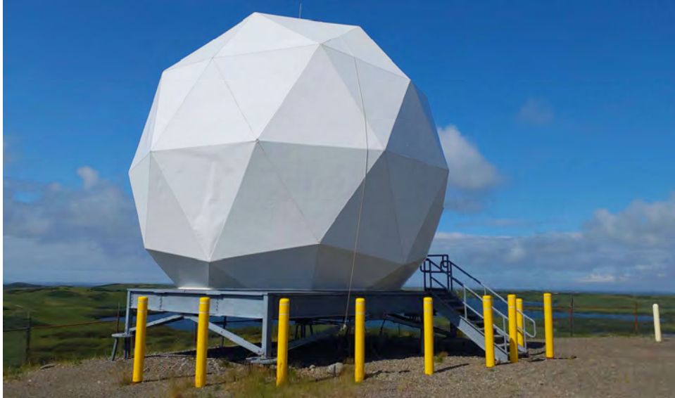
Photograph 3: Satellite communications receiver transmitter. View west.
