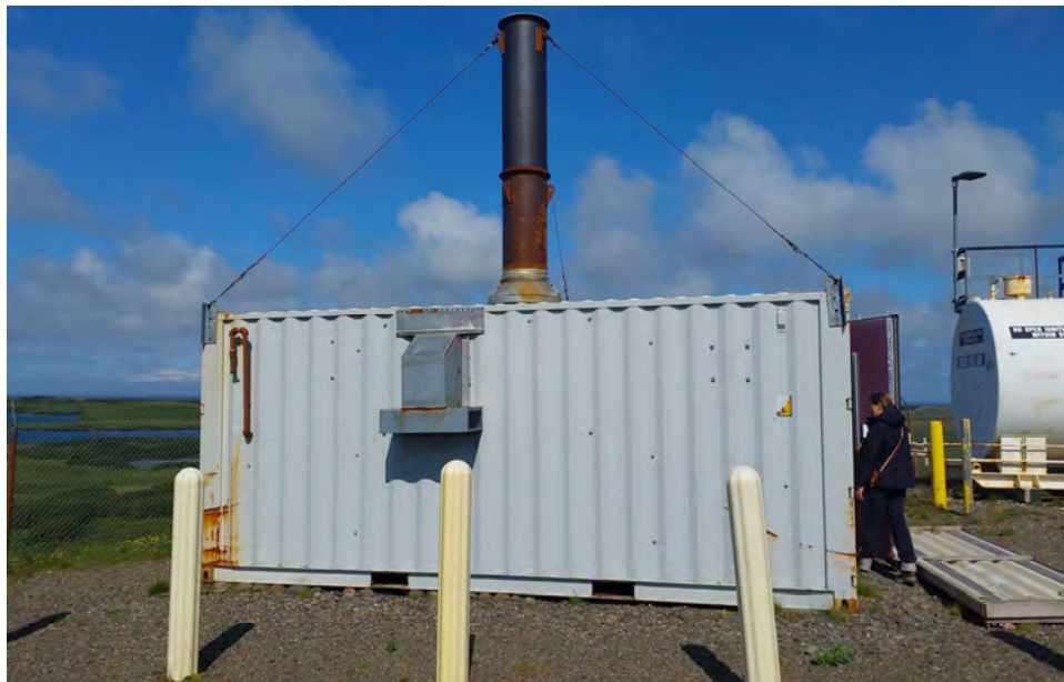
Photograph 8: Non-operational incinerator shed exterior. View north.
