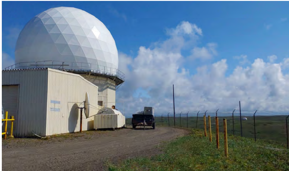
Photograph 2: Radar dome with FAA site in background. View east.
