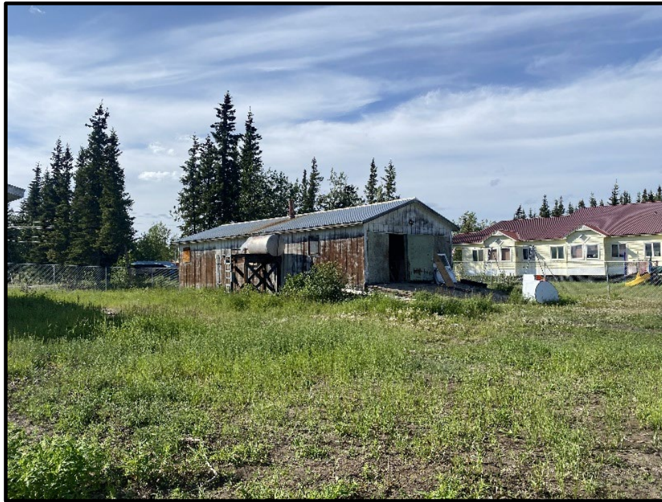
Photo 3: Looking northwest toward Shop Building, with new Cruikshank School in background.
