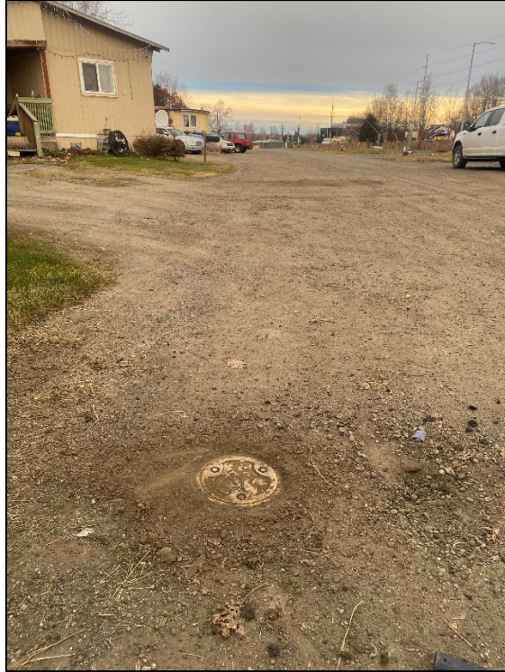
Photograph 7: View looking north. MW-125 after being dug out in relation to the rest of the trailer park.
