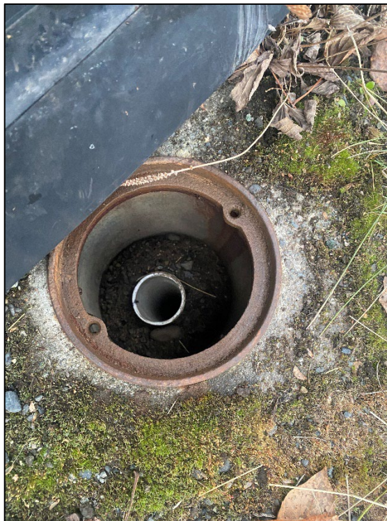
Photograph 4: View looking down. MW-123 opened with well cap off.
