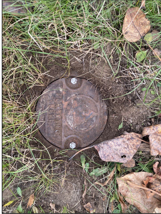
Photograph 11: View looking down. MW-127 closed after being cleaned.
