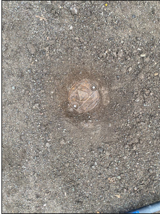
Photograph 5: View looking down. MW-124 closed after gravel covering it was removed.
