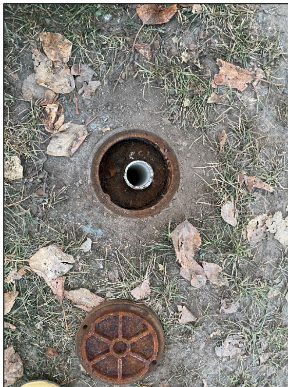
Photograph 14: View looking down. MW-128 opened with well cap off.
