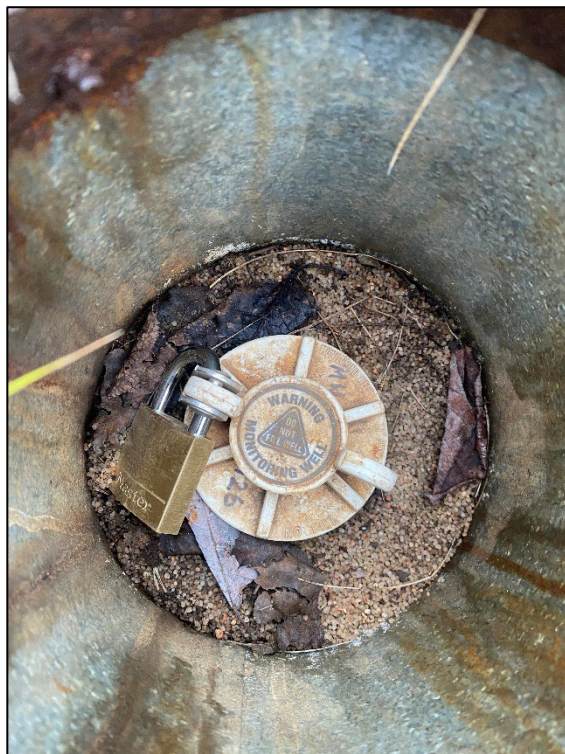
Photograph 10: View looking down. MW-126 opened with new lock installed on well cap. Shows high sand level.
