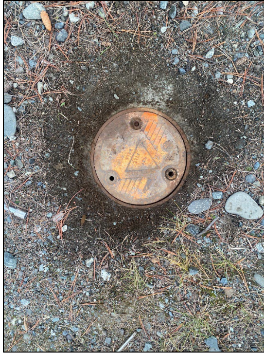
Photograph 15: View looking down. RW-1 closed and cleaned.
