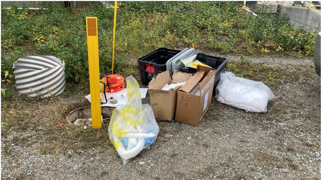
**Photo 4:** Product recovery at MW-1. Note sorbent socks saturated with an emulsion of water and product contained in the oily waste bag (September 8, 2022).
