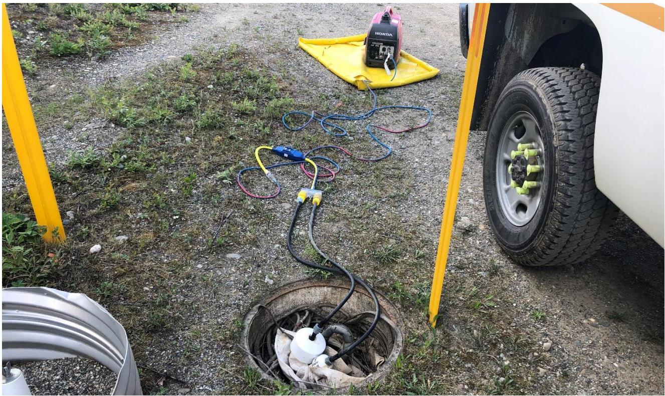
**Photo 1:** Thawing at MW-1 using two heat traces powered by a portable generator (June 7, 2022).
