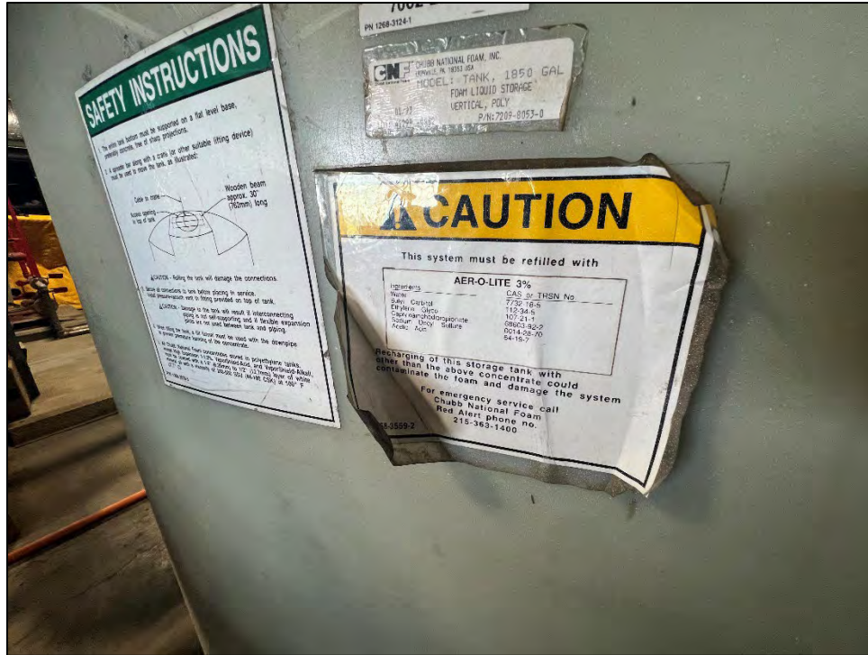
Photograph 34: View close up. Contents of the fire fighting foam AST and warning labels.
