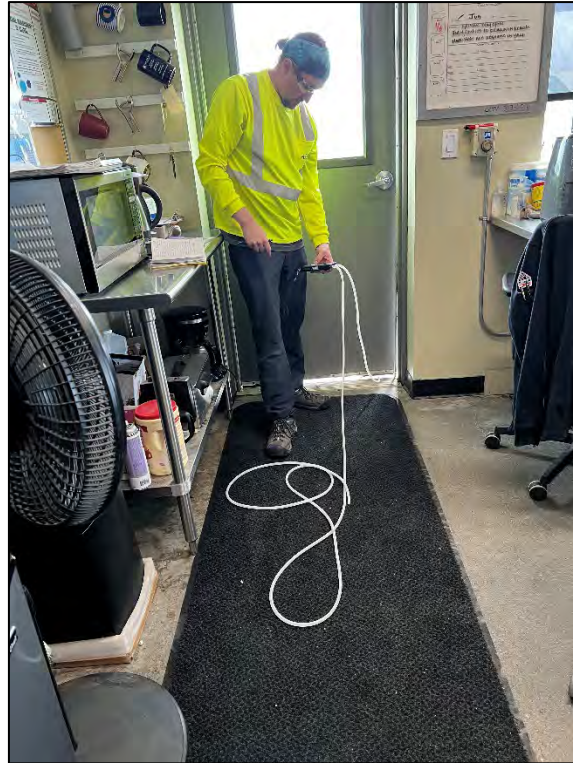
Photograph 40: View looking west. Collecting manometer readings at the west side of the office.
