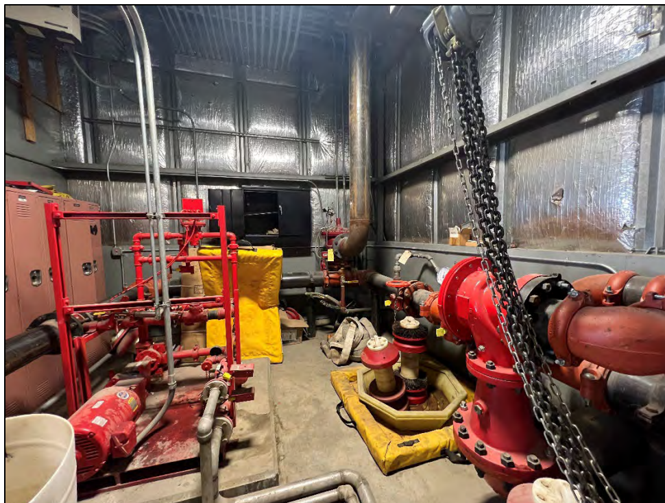
Photograph 31: View looking north. Northeast corner of the garage area.
