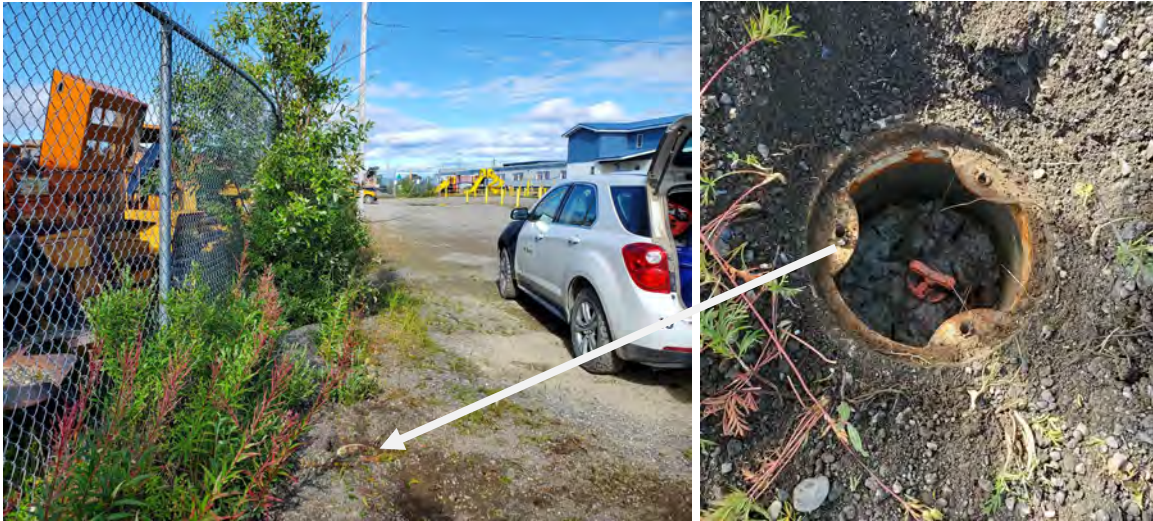
Photo 7: Monitoring Well MW2 located in a parking lot near the fence line. facing northwest. (August 15, 2022)
