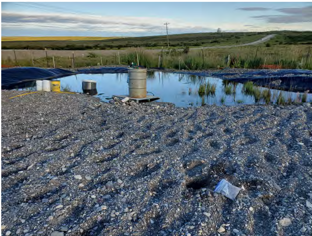
Photo 4: KIC Landfarm: GAC system after recent rainfall event. facing southeast (August 15, 2022)
