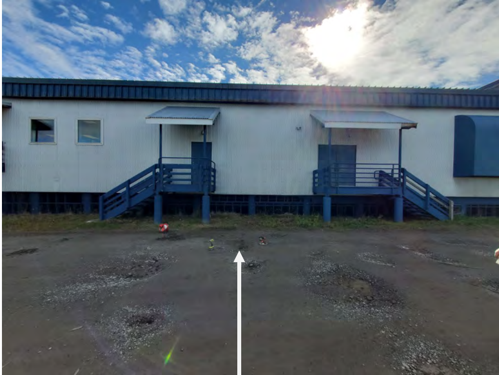
Photo 11: Monitoring Well MW6 located in a pothole along the school backroad. facing southeast. (August 15, 2022)
