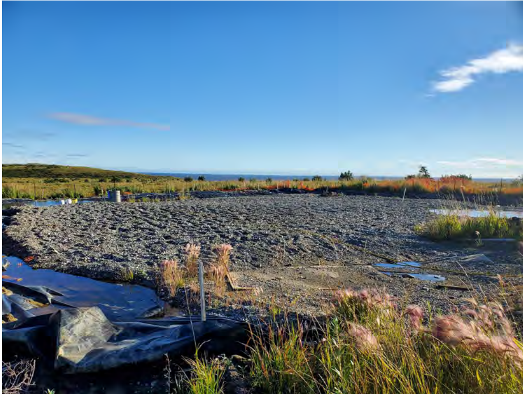
Photo 1: KIC Landfarm: 2020 soil cell in center. 2019 soil cell right of the centerline. GAC filtration system in back left corner. facing south (August 14, 2022)
