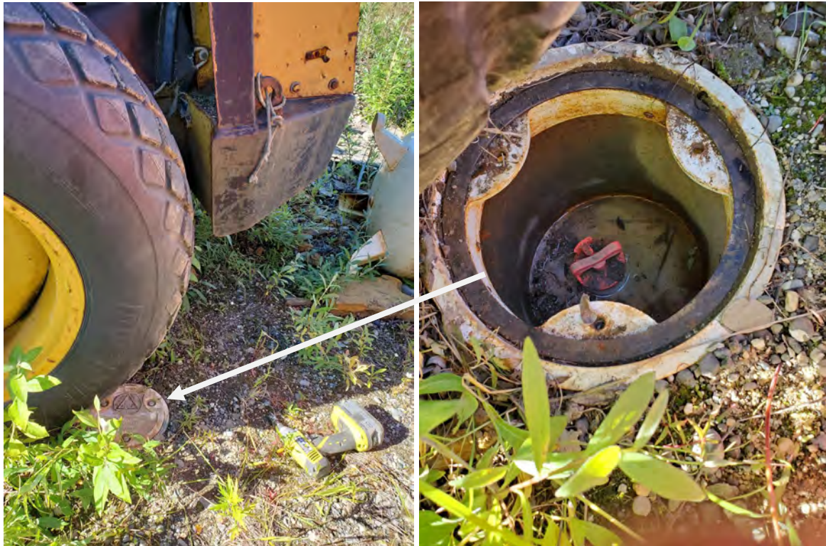
Photo 16: Monitoring Well MW10 located underneath a tire. (August 15, 2022)
