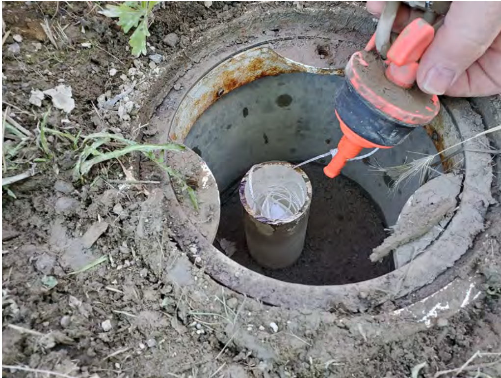
Photo 6: Monitoring Well MW1 had a 3-foot long by 2-inch diameter sorbent sock placed downhole and tied off to the well plug. (August 15, 2022)
