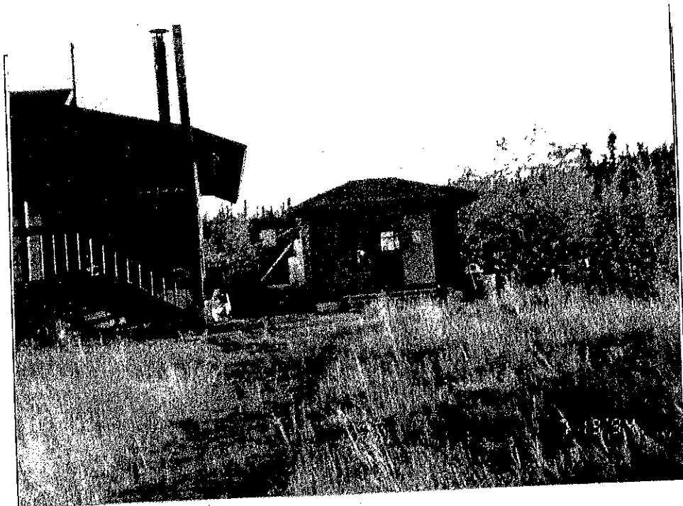
1) Lime Village School and generator shack.
