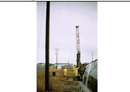
(26) Overhead Power Lines
