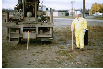
(16) Sample Point GV06, Moved Due to Overhead Communication Lines
