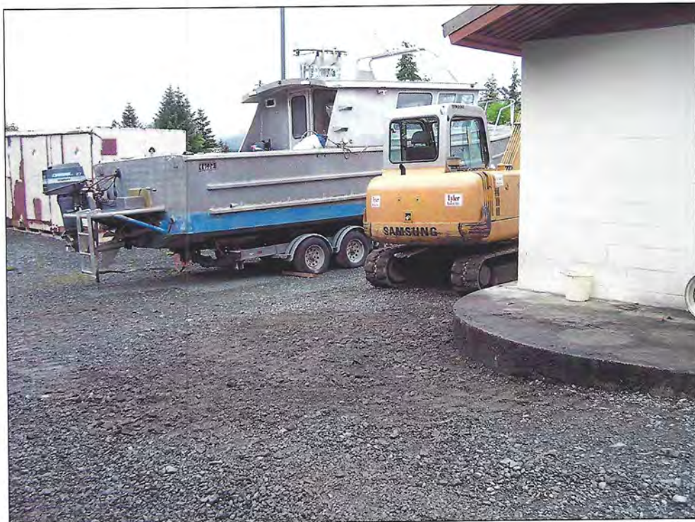
Photograph #2 Spill/excavation site after backfilling and grading. Excavator used for soil removal is along side building; view south (6/29/05).
