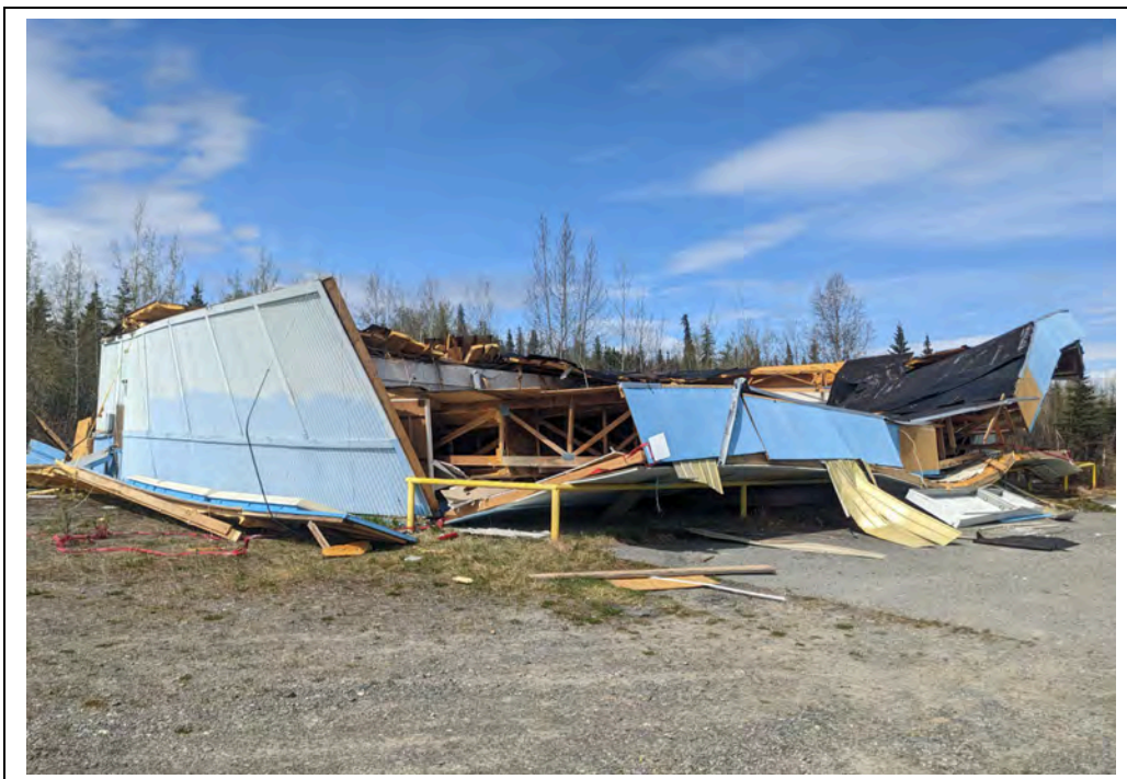
Photo 1: The former Sterling ZipMart convenience store building after collapsing under snow load, looking northwest. The electric meters were on the steel cabinet that has pulled away from the wall leaving an unpainted area at the far left. The lighter colored cabinet remaining on the wall is the telephone connection. (May 23, 2023)
