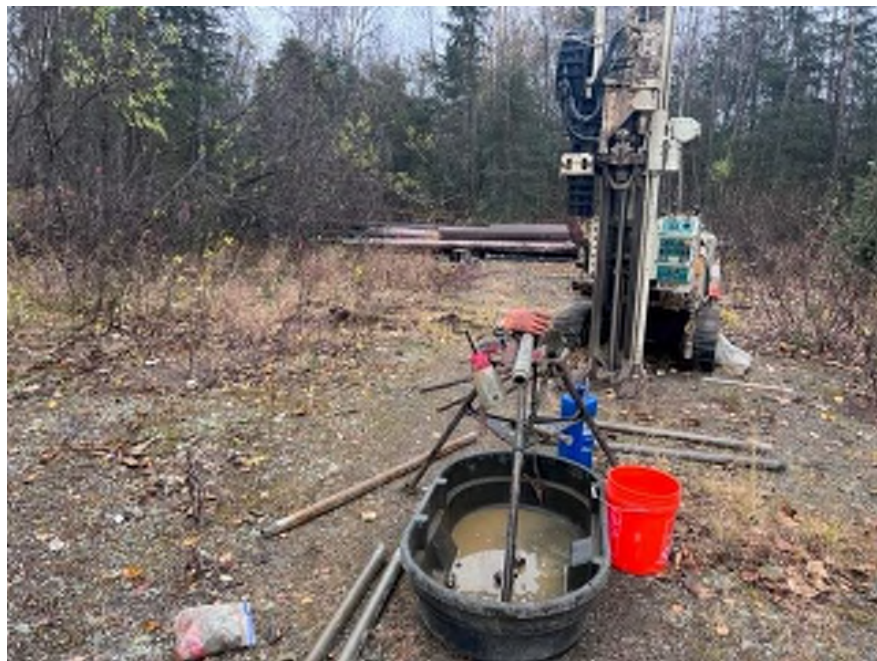
Photo 4, October 12, 2023 – Installing soil boring at Abandoned Diesel Tank Farm, looking southwest.
