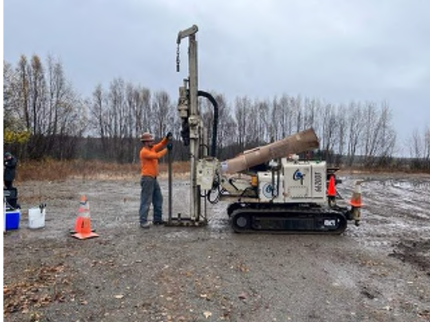
Photo 7, October 13, 2023 – Reinstalling temporary monitoring well 224-13-4, looking southeast.
