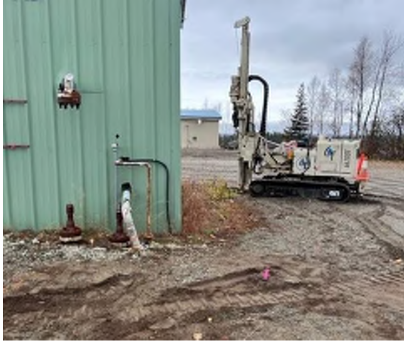
Photo 9, October 13, 2023 – Installing soil boring at 221-23, looking southeast.
