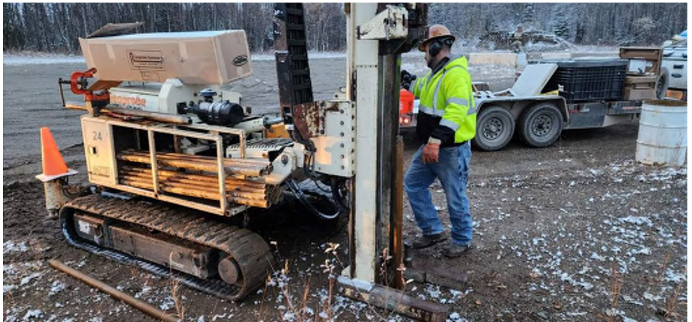
Photo 2, October 12, 2023 – Installing temporary groundwater monitoring well 224-13-4, looking southwest.
