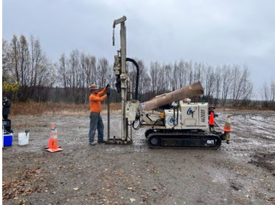
Photo 7, October 13, 2023 – Reinstalling temporary monitoring well 224-13-4, looking southeast.
