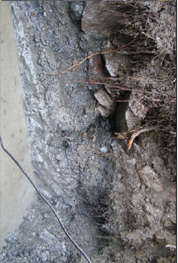
Driveway Excavation Uphill Sump Hole
