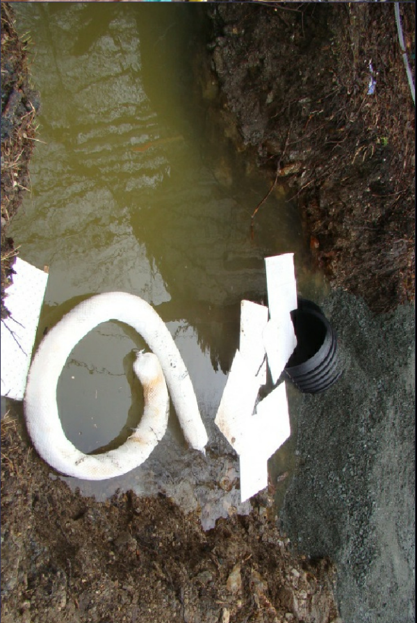
Driveway Culvert Uphill Sump Hole
