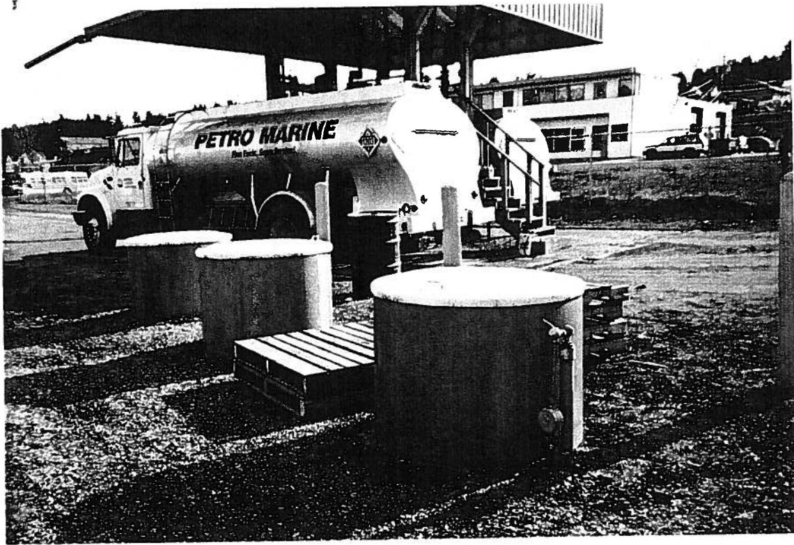
Figure 15. Oil/Water Separator
