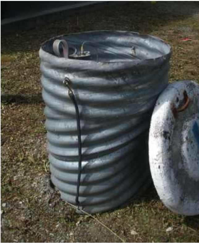
Photo 3: Outfall of oil water separator
