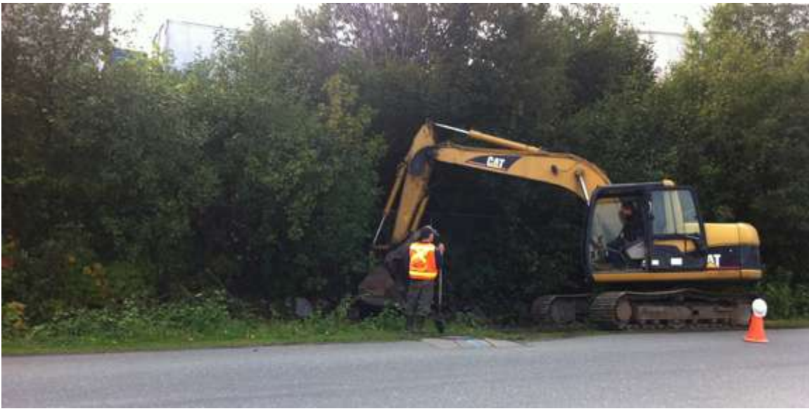
Photo 19: Test Pit #3 was placed adjacent to sewer access.
