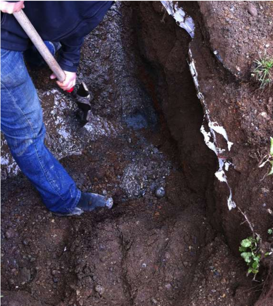
Photo 10: Test Pit #1 encountered groundwater atop clay at 4 feet below ground surface.
