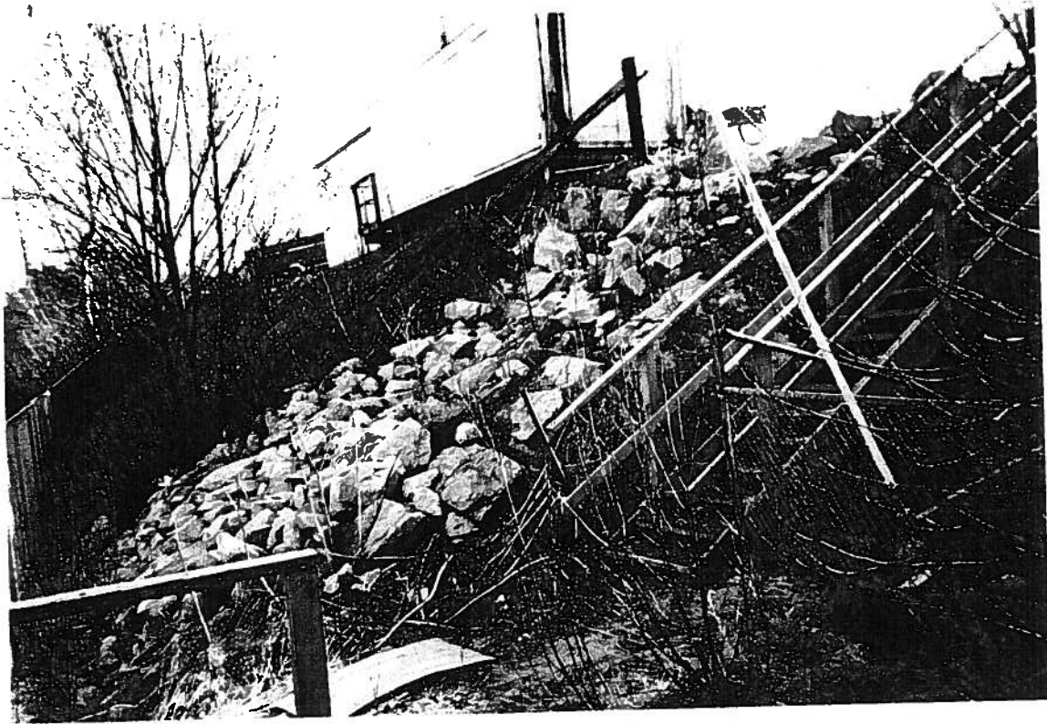
Figure 19. Shotrock on western edge of Petro Marine Haines property
