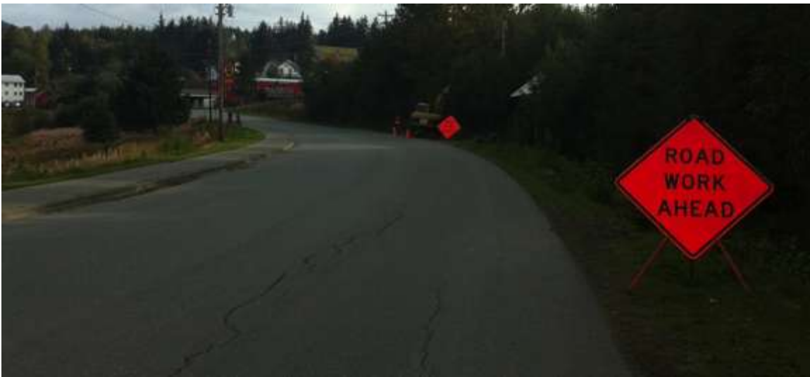
Photo 18: Proper signage was placed during fieldwork event.
