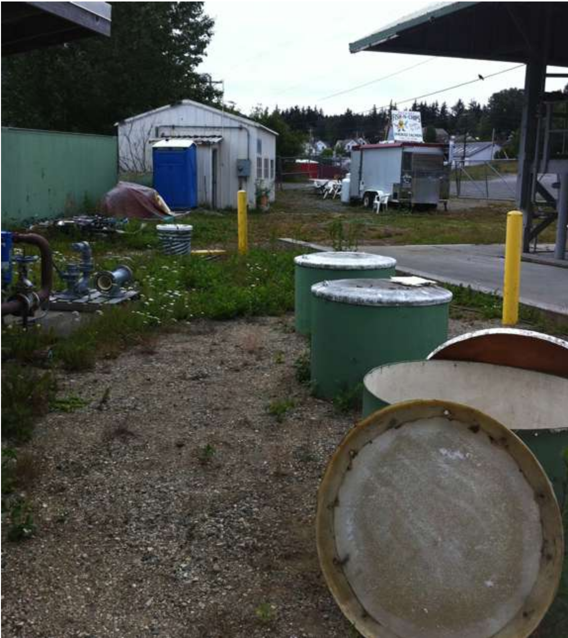
Photo 1: Truck rack photo right. Three green vessels provide access to Oil Water Separator system (OWS) with the first tank featuring 4 inches of fuel prior to removal of 20 drums of mixed oil and water in 2011. Vertical culvert pipe left of far yellow safety post is the subsurface outfall of the system.
