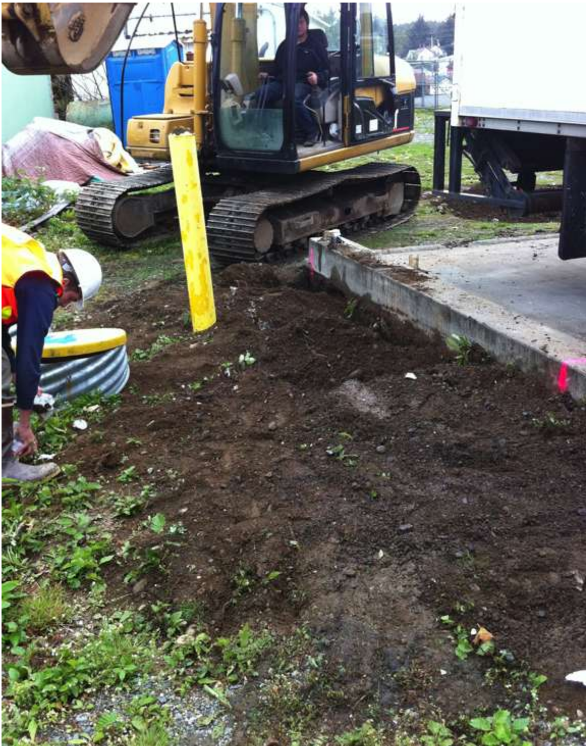
Photo 12: Test Pit #1 was closed and the disturbed soil was compacted to minimize impacts to the property. Buried lines were documented with pink spray paint on the truck rack.
