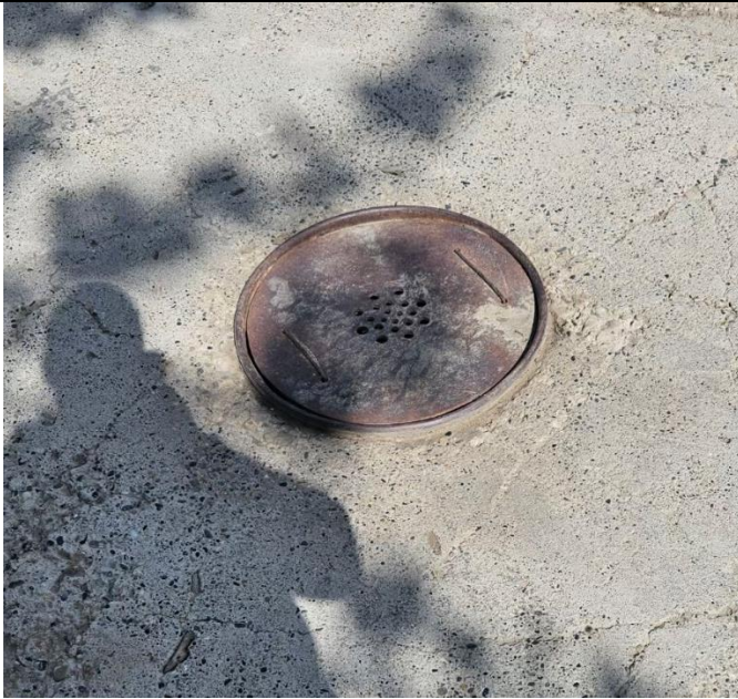
Drywell lid before sealing and covering.
