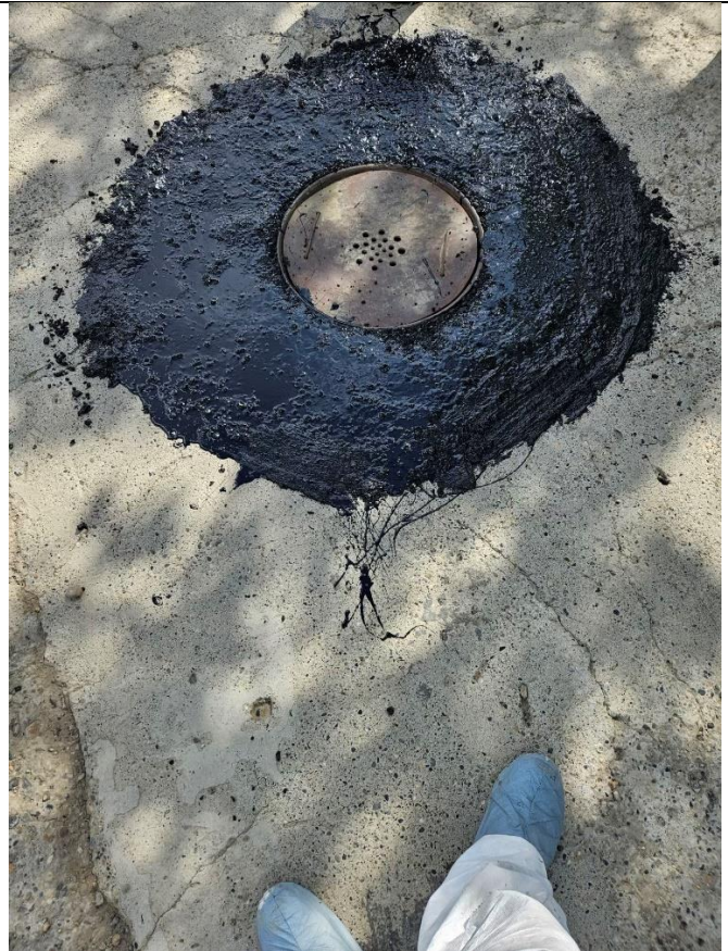
Sealing tar brushed on top of the asphalt.
