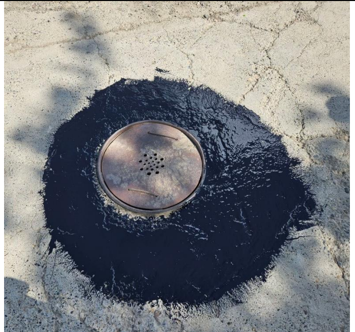
Sealing tar brushed around the drywell on cleaned concrete.
