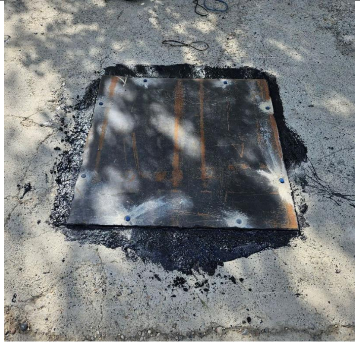
Additional view of steel Cap Plate.
