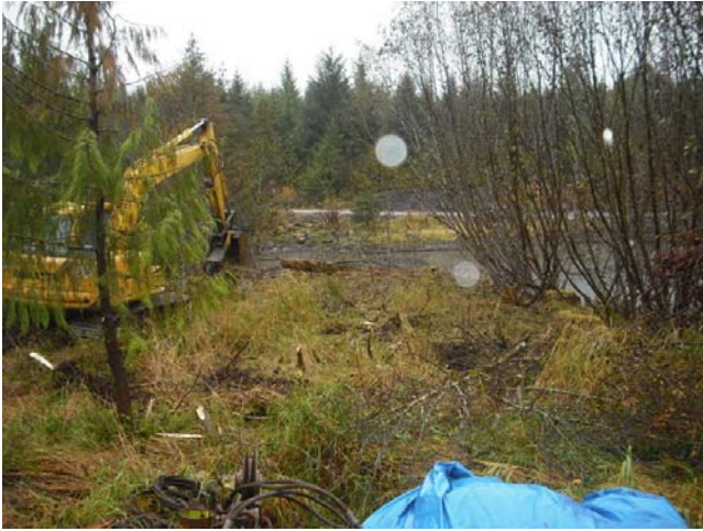
Photograph 1 ~ Commencement of Test Pit 1 Excavation (facing north-northwest)
