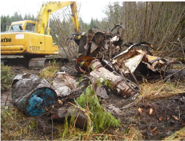
Photograph 3 ~ Drums, Automobile Parts, and Various Metals Uncovered in Test Pit 1.
