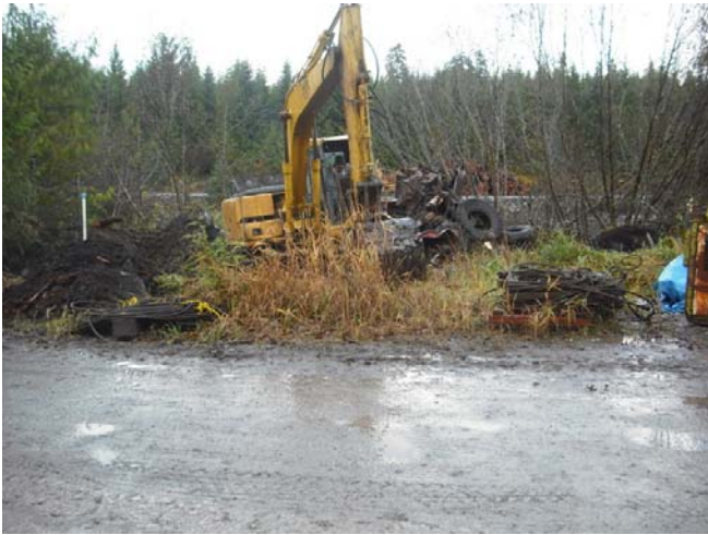
Photograph 7 ~ Commencement of Test Pit 3 Excavation (facing north-northwest)
