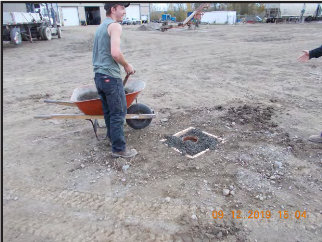
PHOTOGRAPH 5: VIEWED SOUTHEAST- INSTALLATION OF CONCRETE TO SECURE WELL MONUMENT
