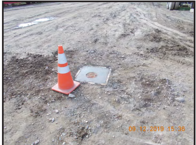
PHOTOGRAPH 6: CLOSE UP VIEW OF WELL MONUMENT SECURED WITH CONCRETE
