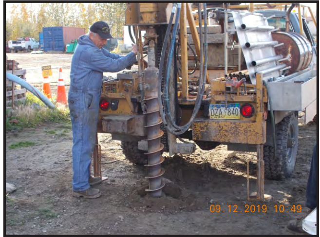
PHOTOGRAPH 2: VIEWED SOUTHWEST- ADVANCING 6" HOLLOW-STEM AUGER TO INSTALL MW-1
