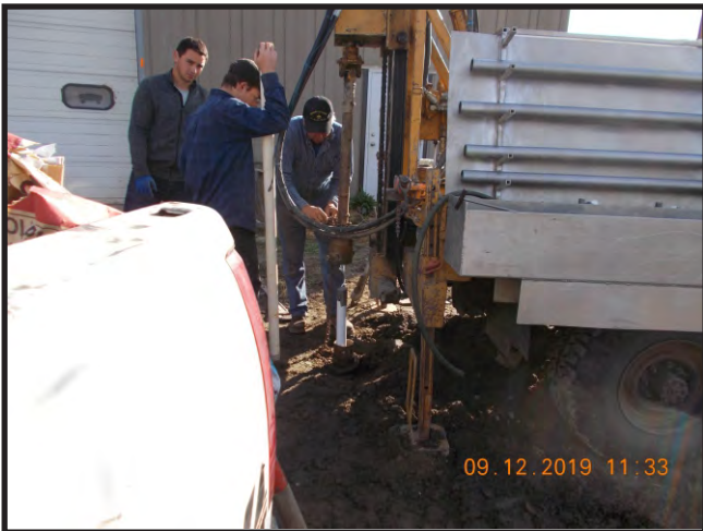
PHOTOGRAPH 3: VIEWED EAST- INSTALLATION OF MW-1 WELL SCREEN AND CASING
