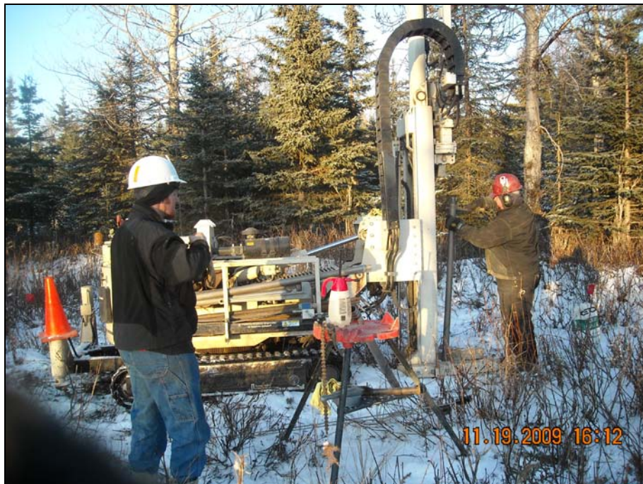
Former Trench Area Burn Pit – Hammer Environmental collecting core samples (View to NW)
