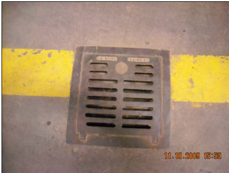
Maintenance Building 55 - Typical floor drain found during building inspection
